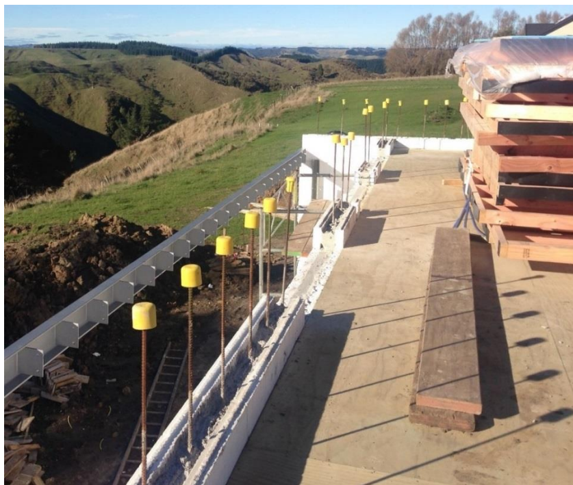
Figure 13: Photo of the junction between the first floor and the walls
