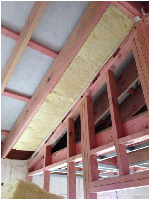
Figure 14: Photo of the insulation in the roof space
