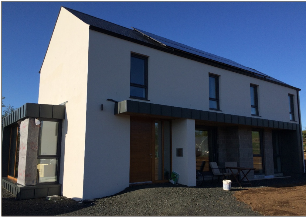
Southern facing elevation with large glazed areas with zinc shading, and the large glazed doors to open plan area recessed further back to reduce summer solar gain. 4kw of PV panels on the roof.
