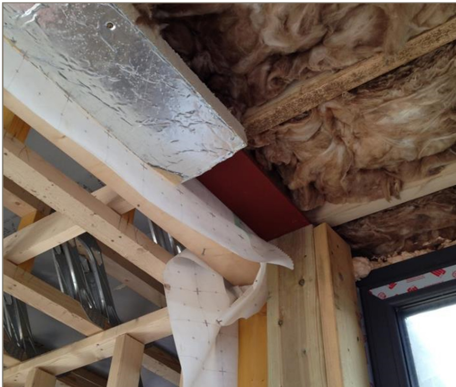
PIR (0.022 w/mK) inside web of the steel beam and around the exterior, in the Sitting Room reducing thermal bridging.
