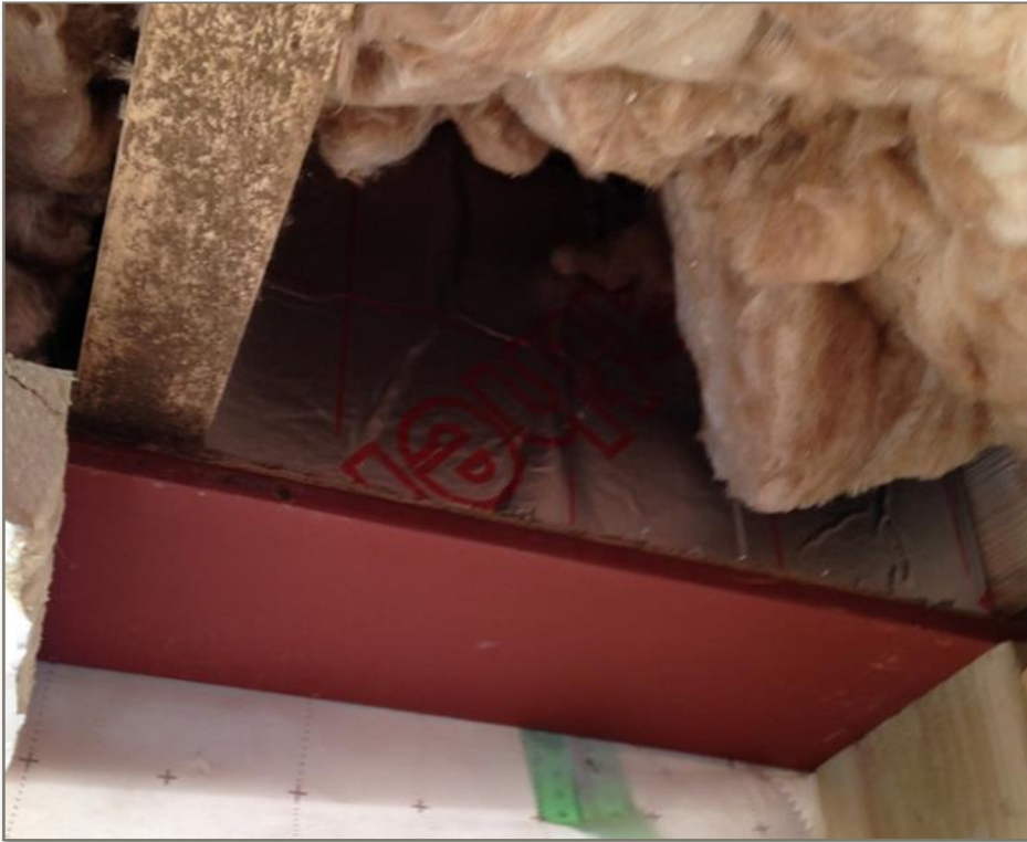
PIR (0.022 w/mK) inside web of the steel beam and around the exterior, in the Sitting Room reducing thermal bridging.
