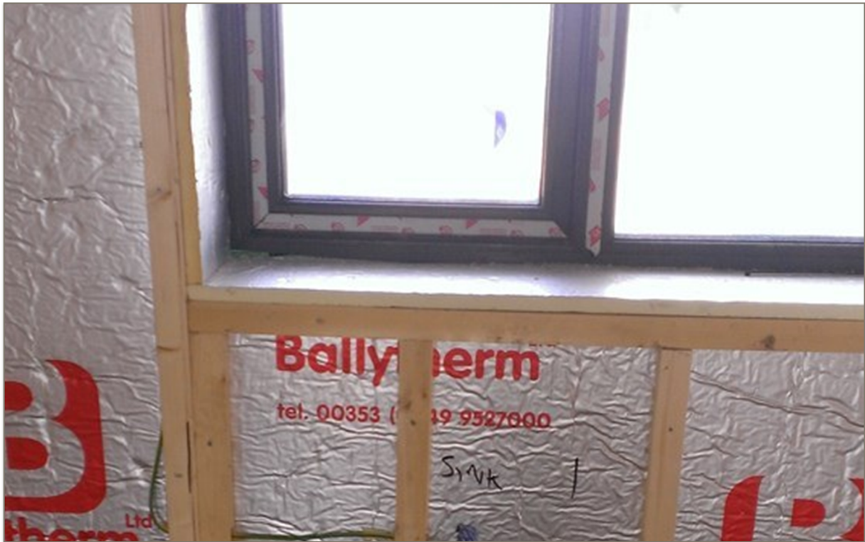
80mm PIR (0.022 w/mK) boards on walls with 25mm PIR (0.022 w/mK) around windows to reduce thermal bridging with service battens in place.
