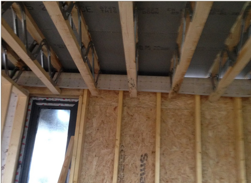
First floor joist hung from wall
