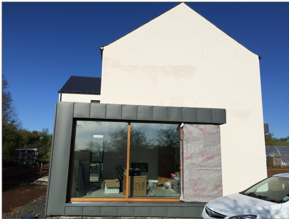
West elevation with projection zinc box, with openable windows in either corner to provide cross ventilation.
