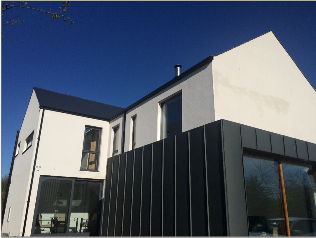
Northern & West elevation, with large doors to the open plan area to provide cross ventilation.
