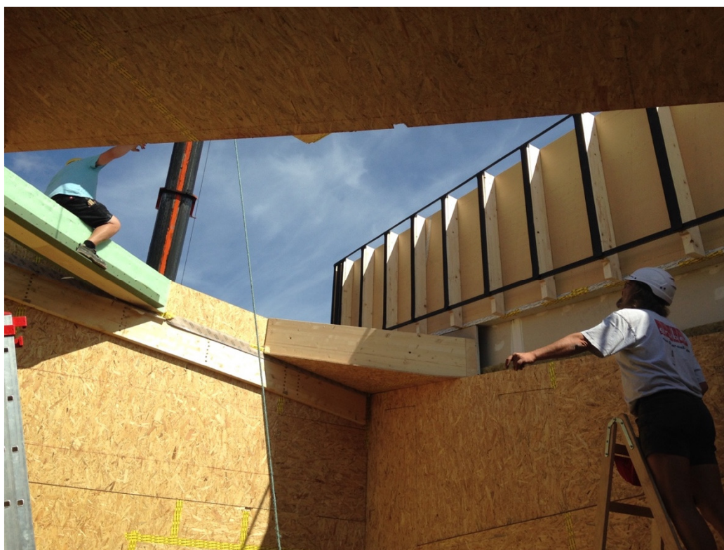
Closing the roof / Dachschliessung
