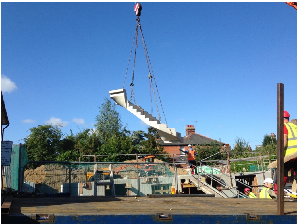
Staircase / Treppe Haus I
