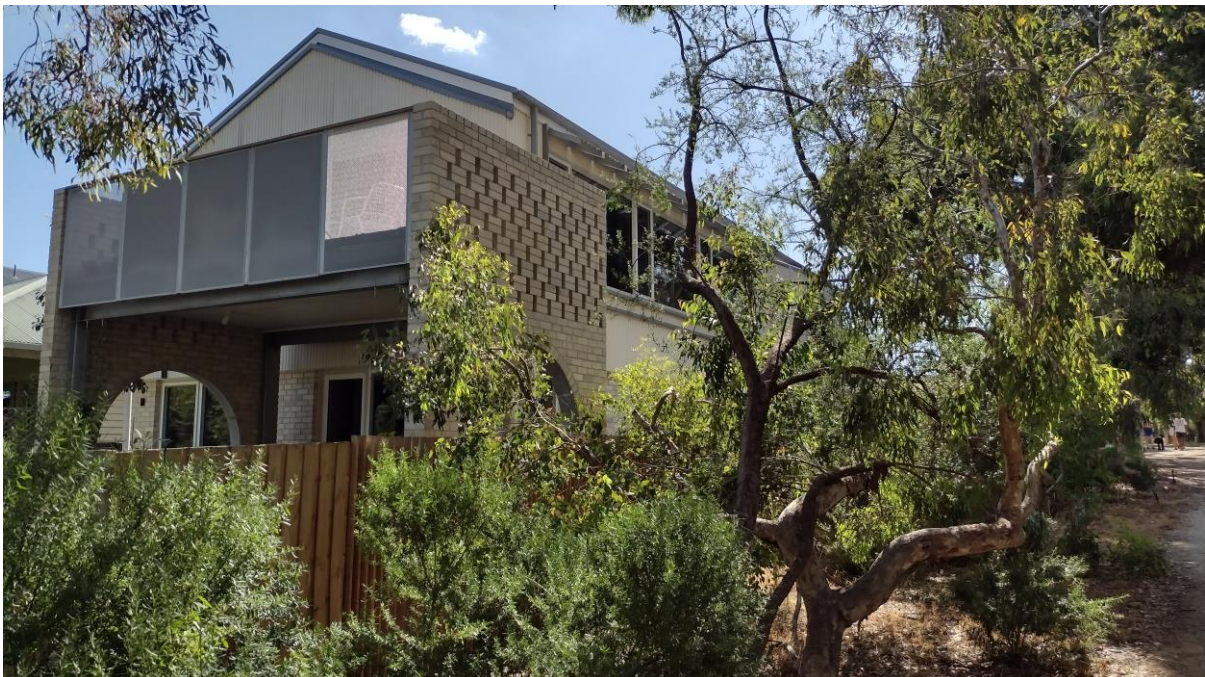
North-East corner of the dwelling, showing shading provided by first floor deck and trees
