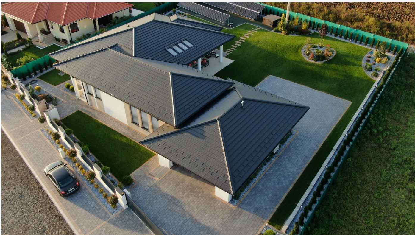
Aerial view of the building from the southeast, with the garage block in the foreground. The solar panel system is visible behind the building.
