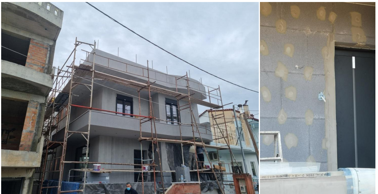
Picture 5. Placement of the exterior insulation of the thermal envelope
