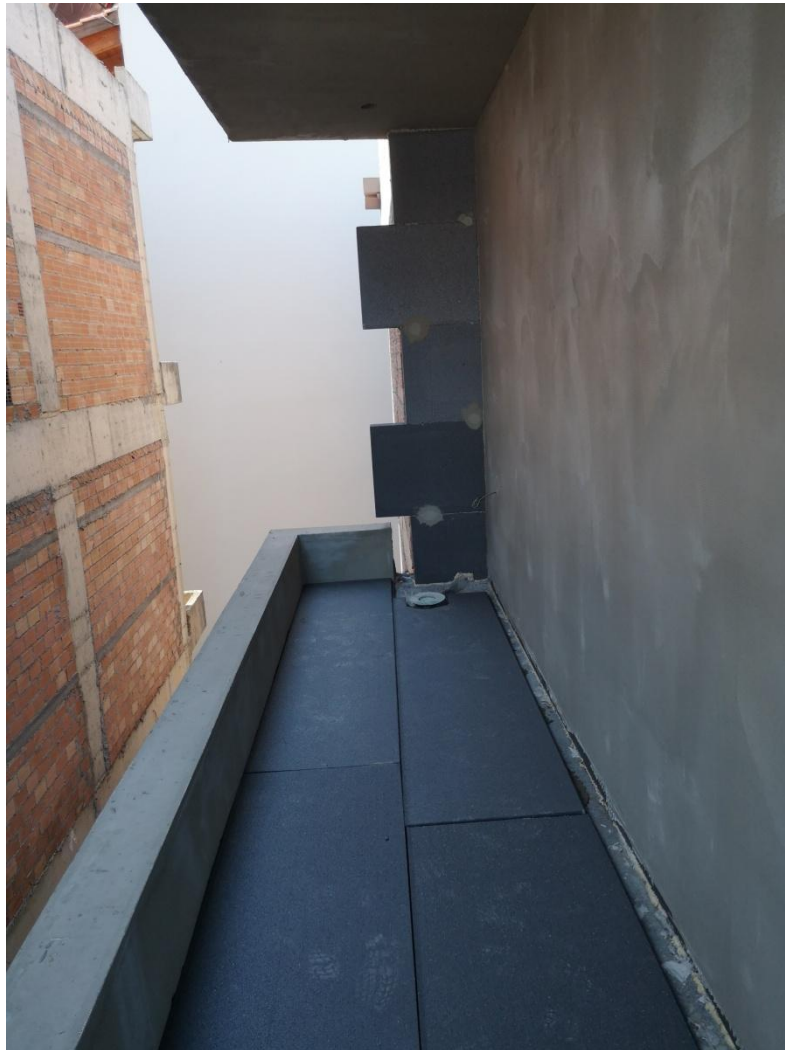
Picture 8. Balcony insulation
