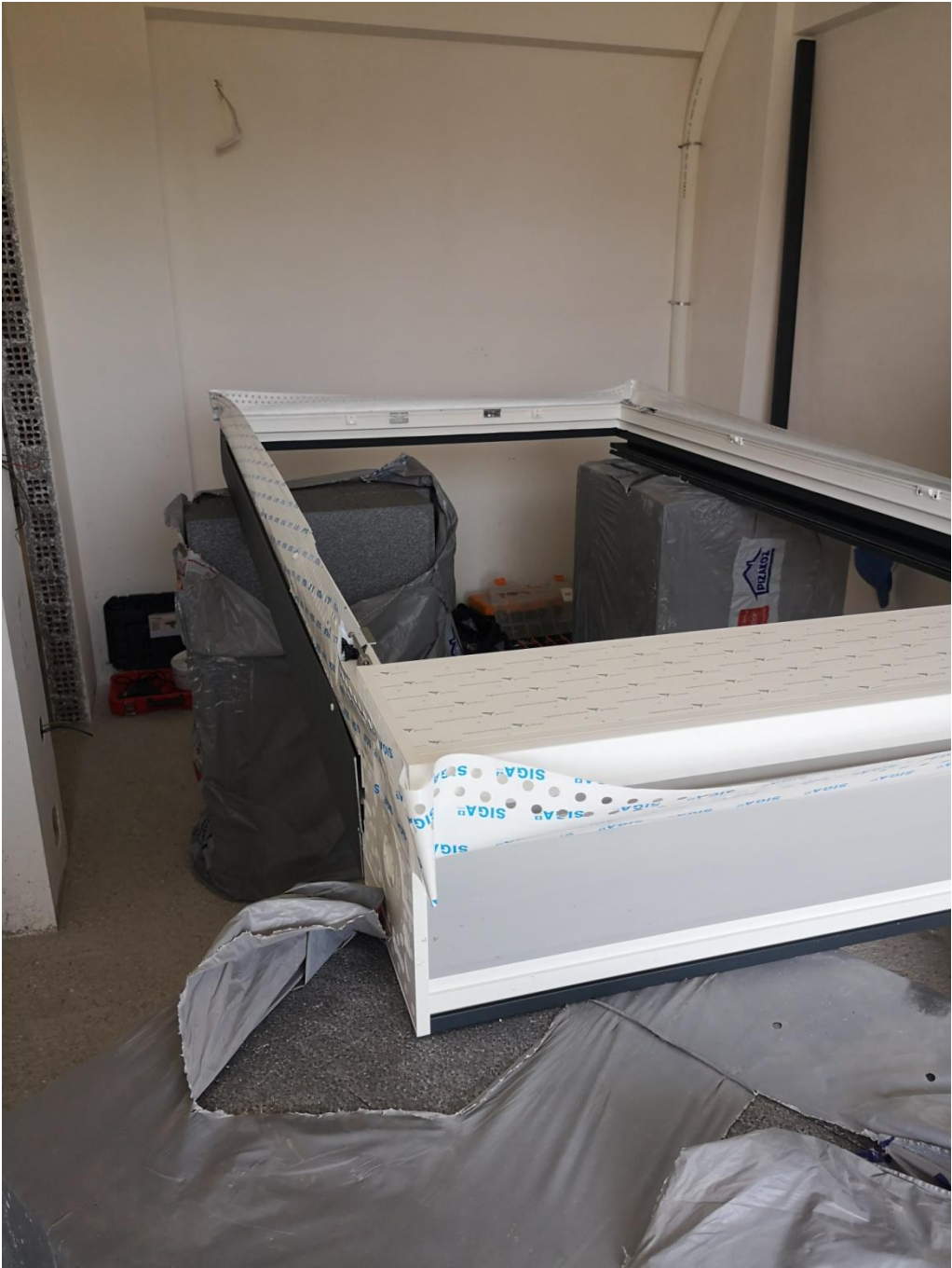
Picture 13. Windows airtight installation
