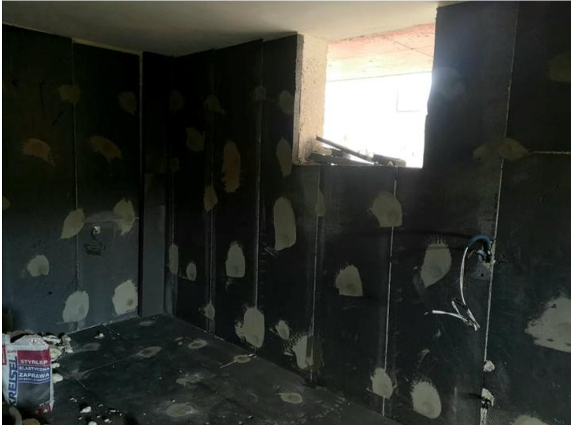
Picture 6. Basement wall and slab insulation
