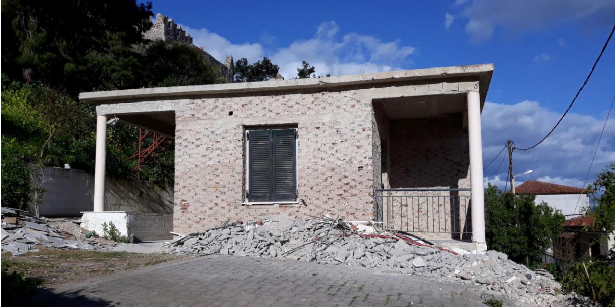
Picture 20: External brick walls renovation.
