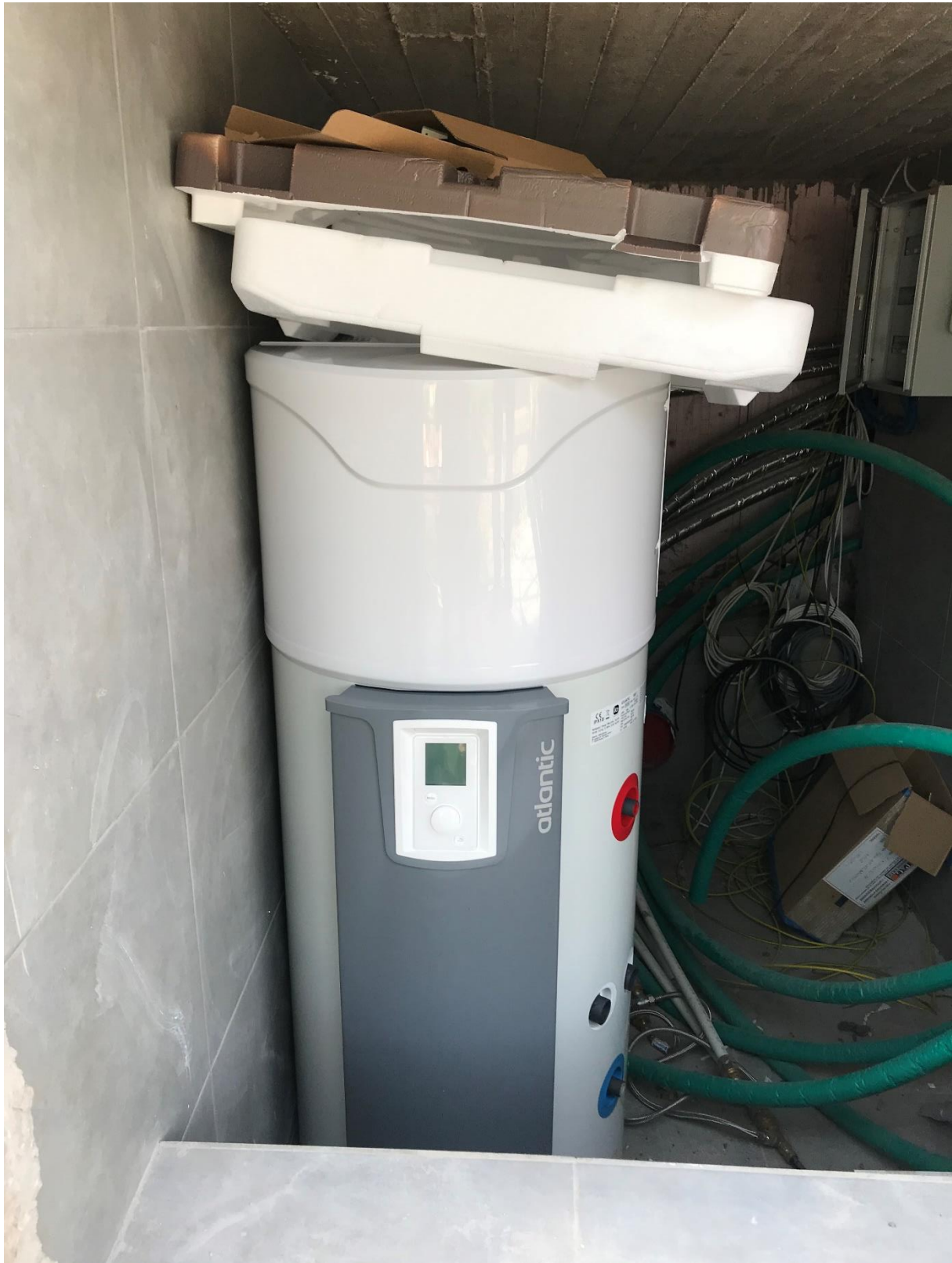
Picture 44: DHW heat pump during installation.
