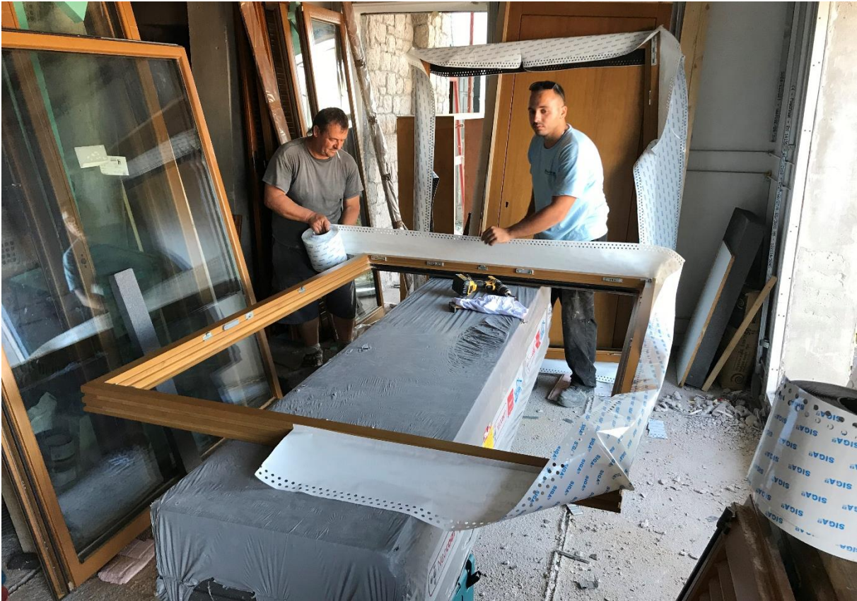
Picture 35: Special tapes applied around the window frame before installation.
