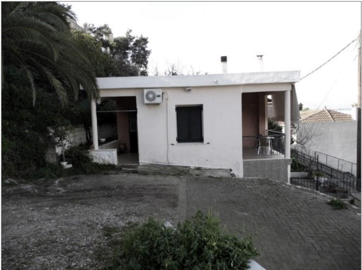
Picture 2: East view of the existing building.
