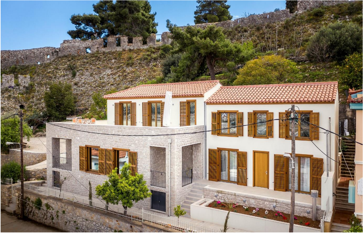
Picture 5: North - West view of the new construction.
