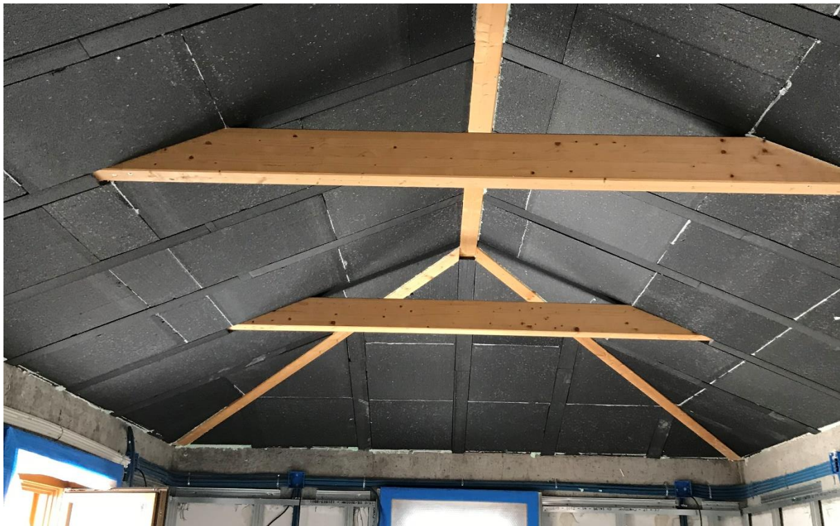
Picture 27: Roof, first floor apartment.
