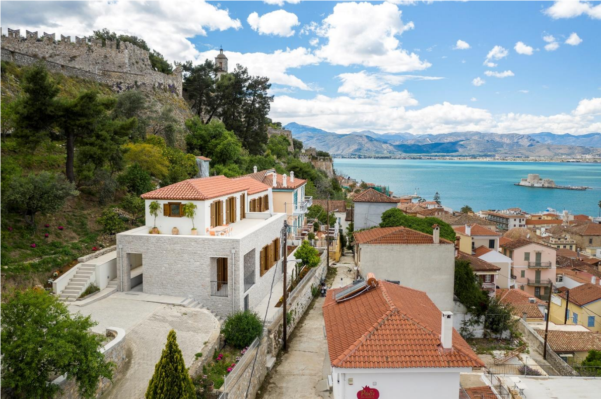
Picture 6: North - East view of the new construction.
