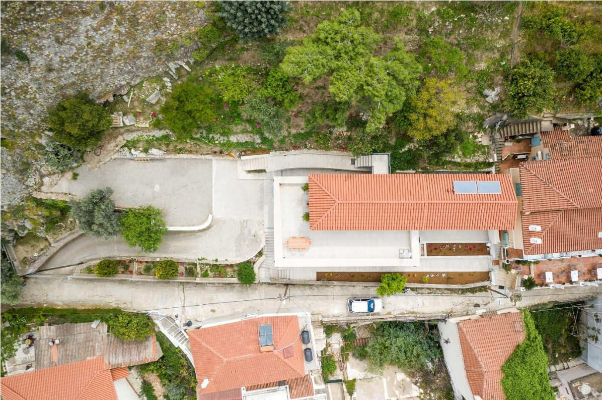
Picture 8: Top view of the new construction.
