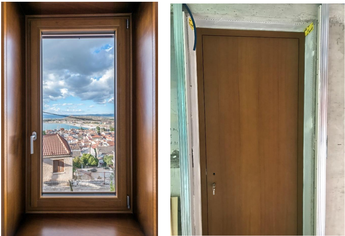
Picture 30: Triple glazed, wooden framed windows and opaque wooden door.
