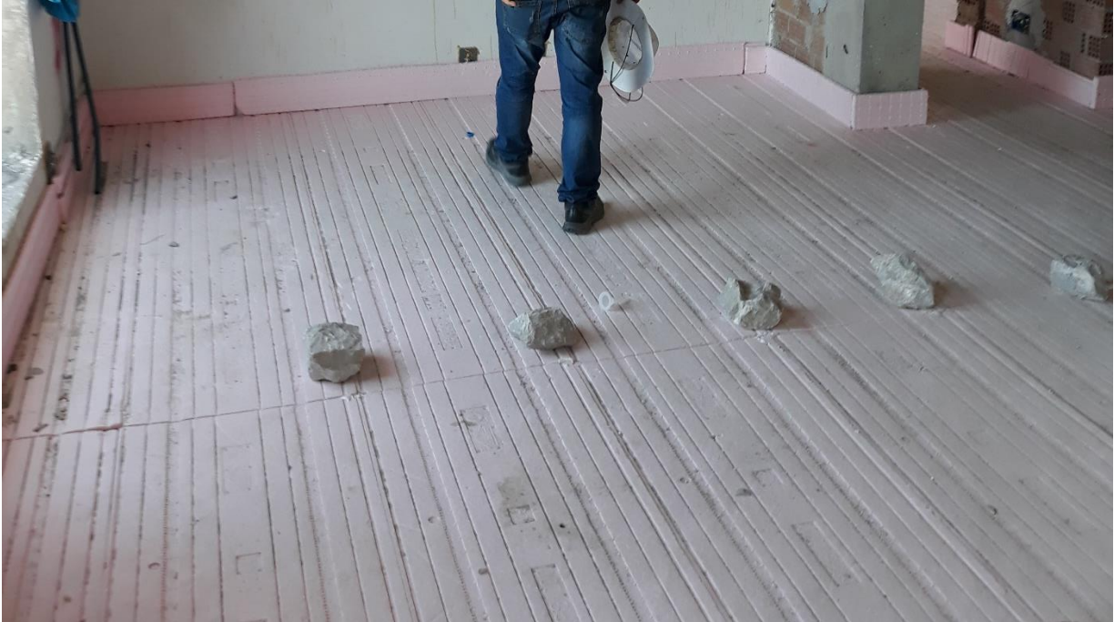
Picture 16: Ground floor insulation, existing building.
