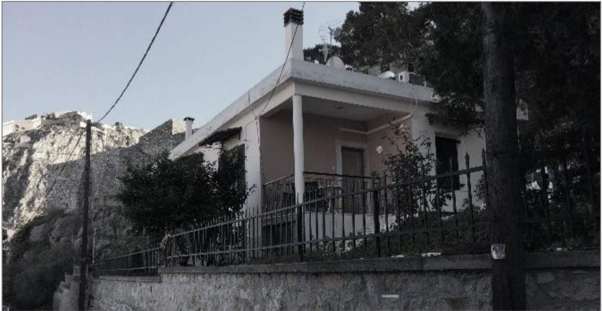
Picture 3: West view of the existing building.
