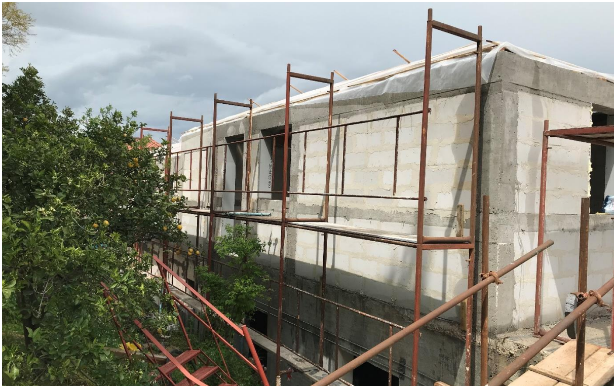
Picture 23: Thermal blocks extension in height, south view.
