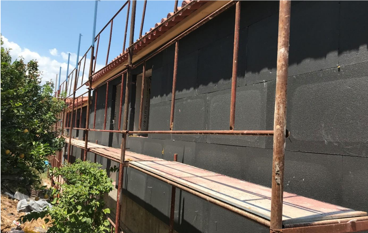
Picture 24: Wall insulation, south view.
