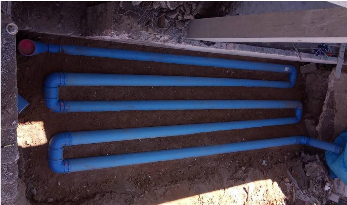
Picture 41: Subsoil heat exchanger during installation.
