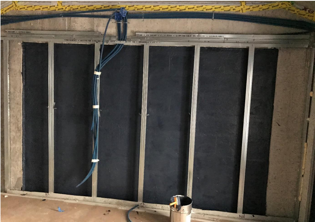
Picture 34: Aerosana, airtight material used on thermal block walls.
