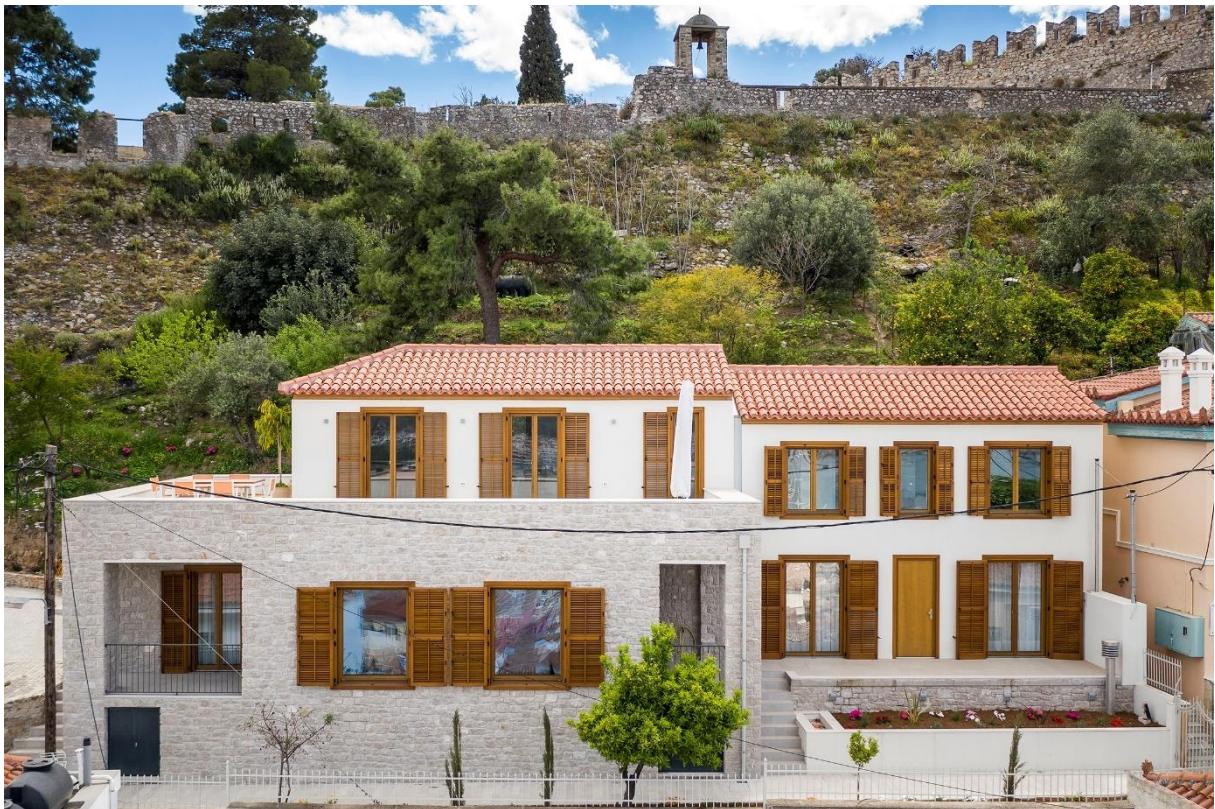
Picture 4: North view of the new construction.
