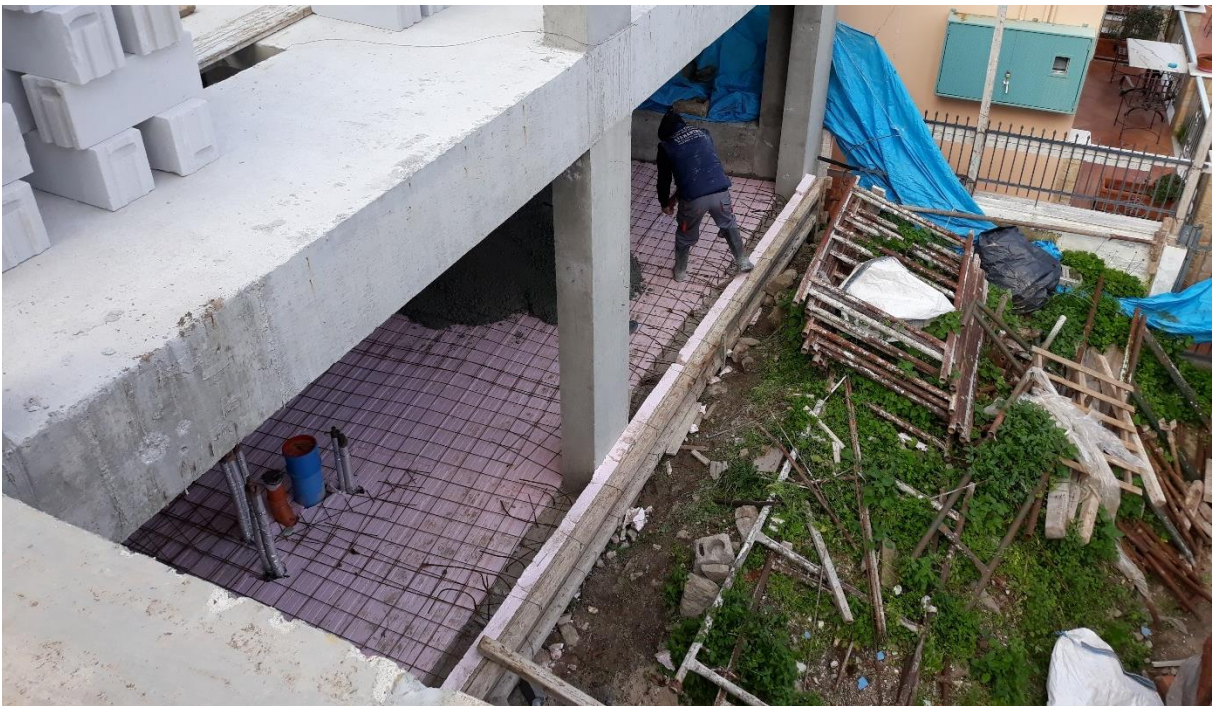
Picture 17: Ground floor insulation, new construction.
