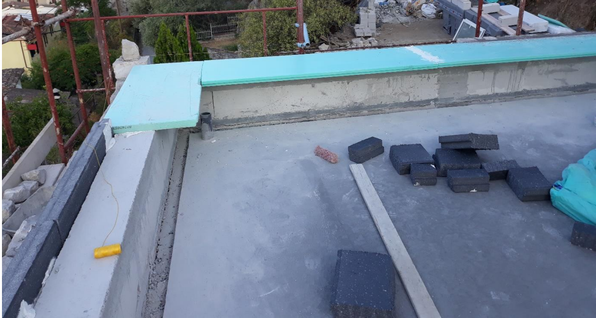
Picture 26: Ceiling, ground floor, existing building.
