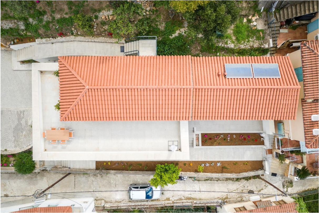
Picture 46: Sollar collectors facing south.
