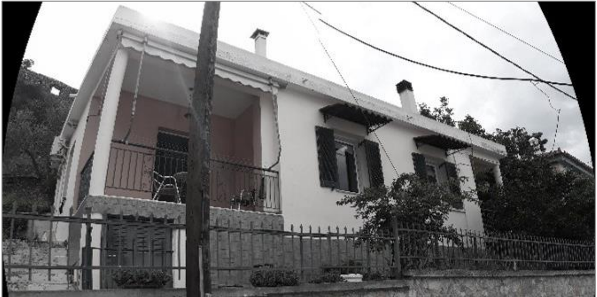
Picture 1: North view of the existing building.
