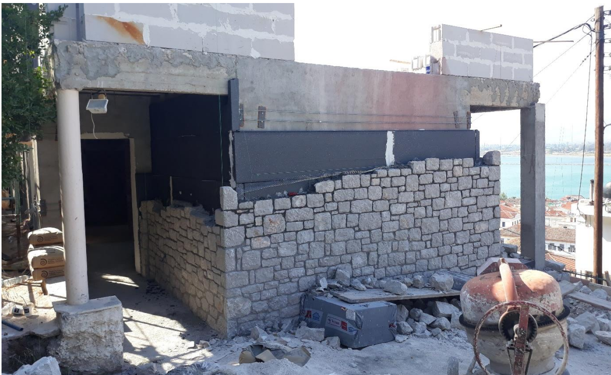
Picture 21: External brick walls.
