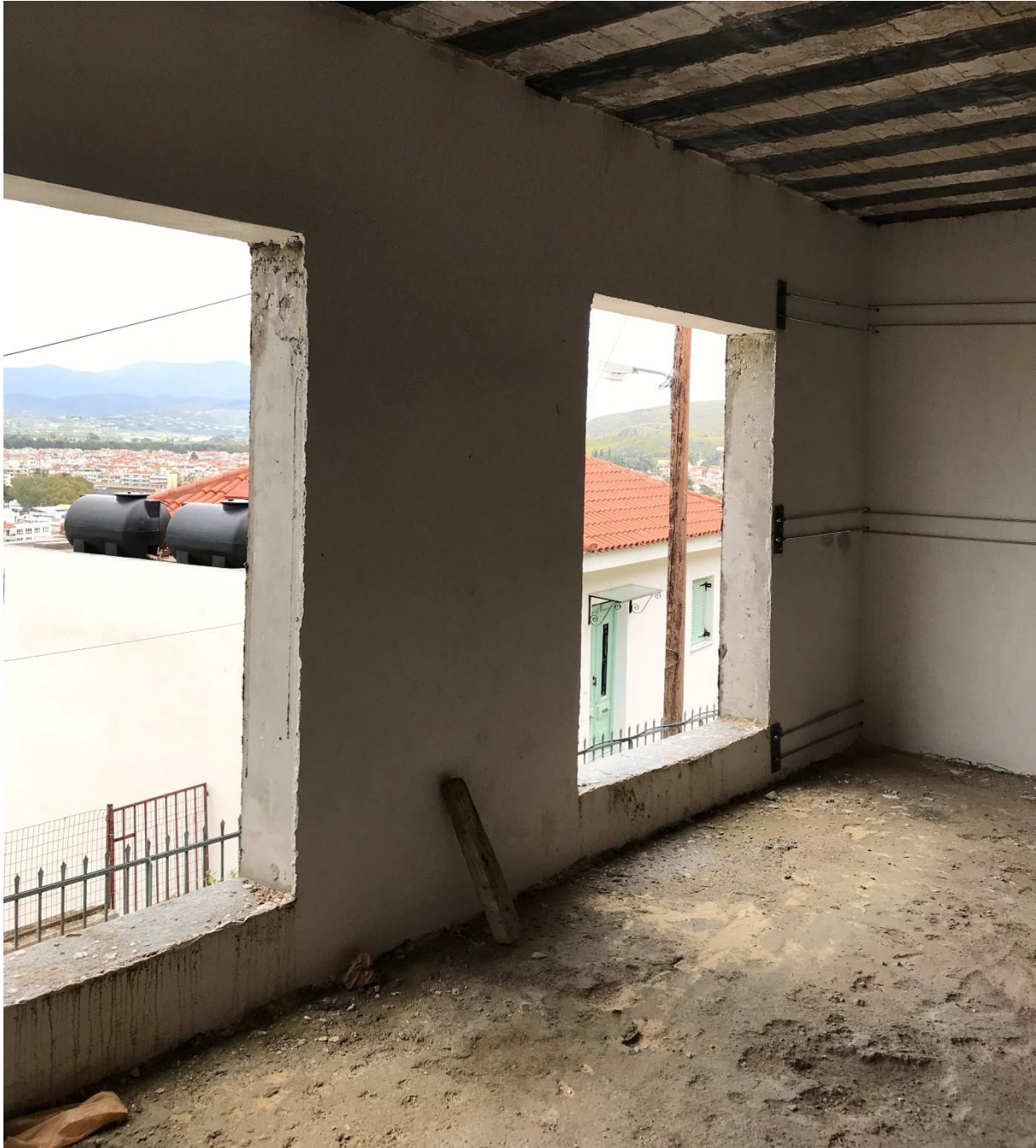
Picture 33: Plaster applied on the brick walls as an airtight layer.
