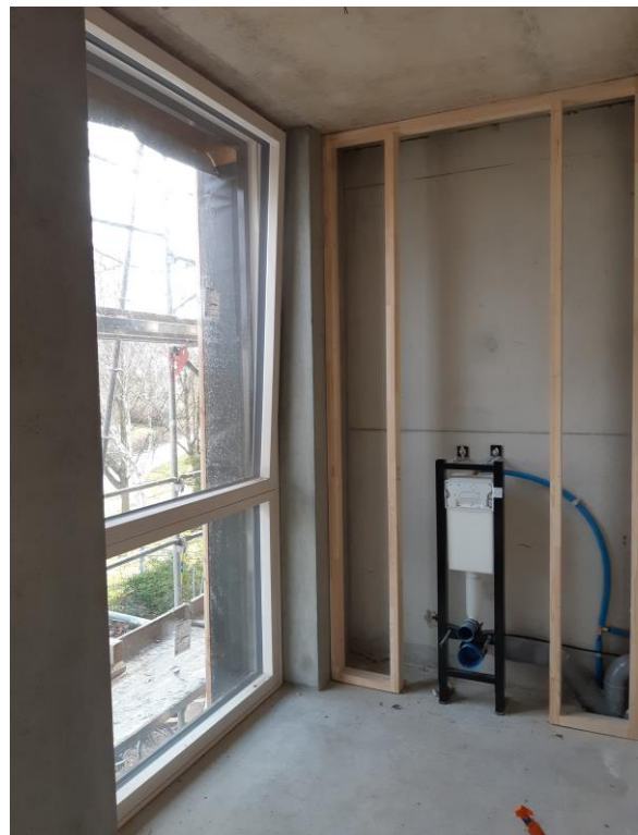
Figure 21 : Photo of window
