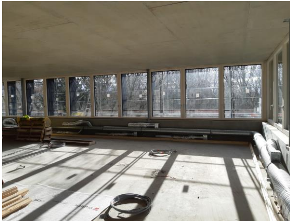
Figure 20 : Photo of windows
