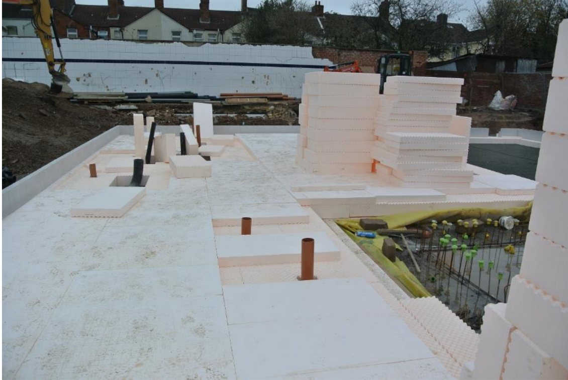
Photo of under floor slab installation. .
