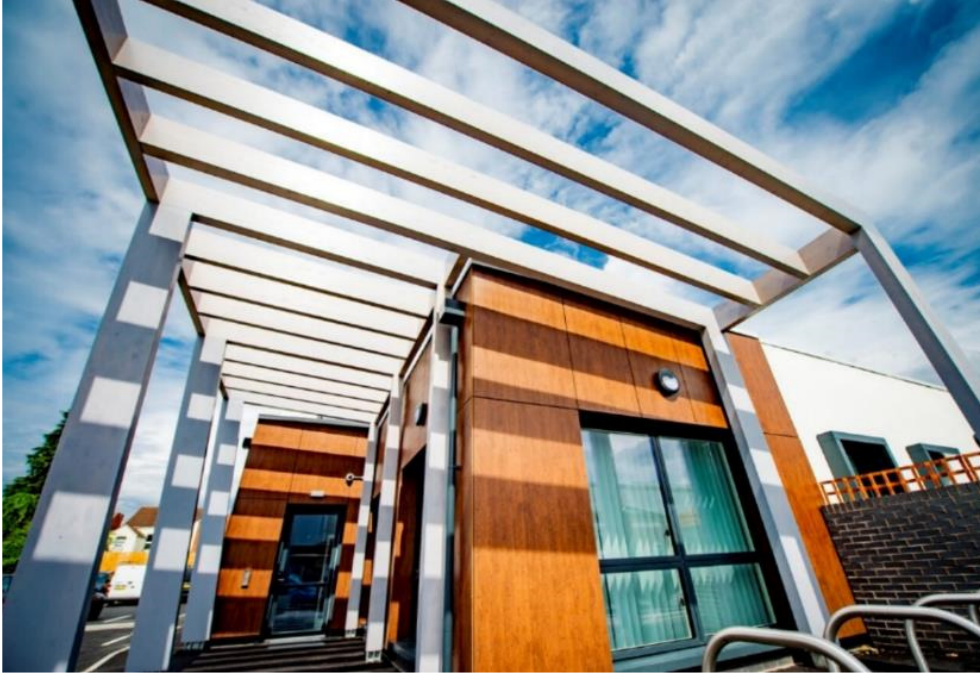
Front (south facing) elevation to Livingstone Road – pergola provides shading to SW and S facing windows to waiting room
