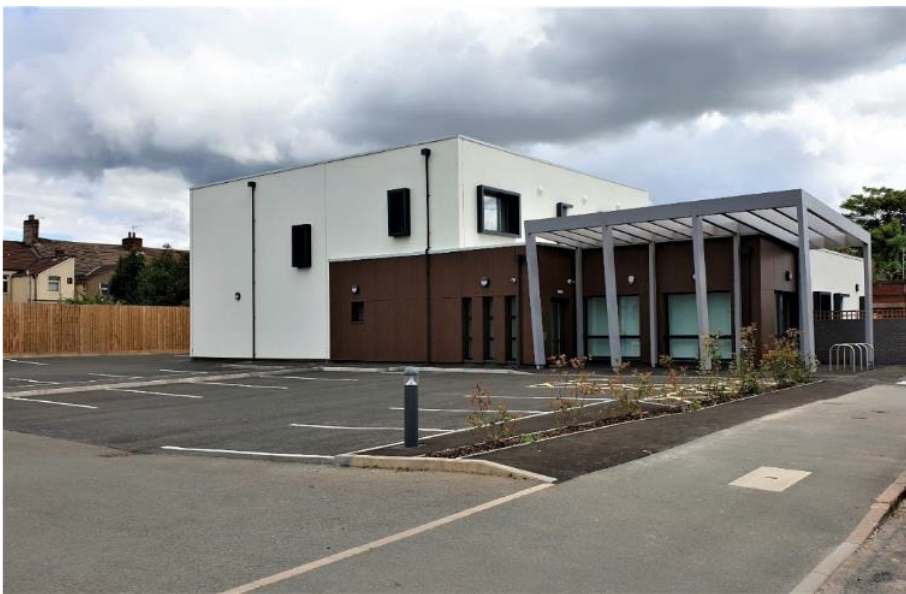
West facing elevation towards car park. Entrance and waiting room at south west corner of the building.
