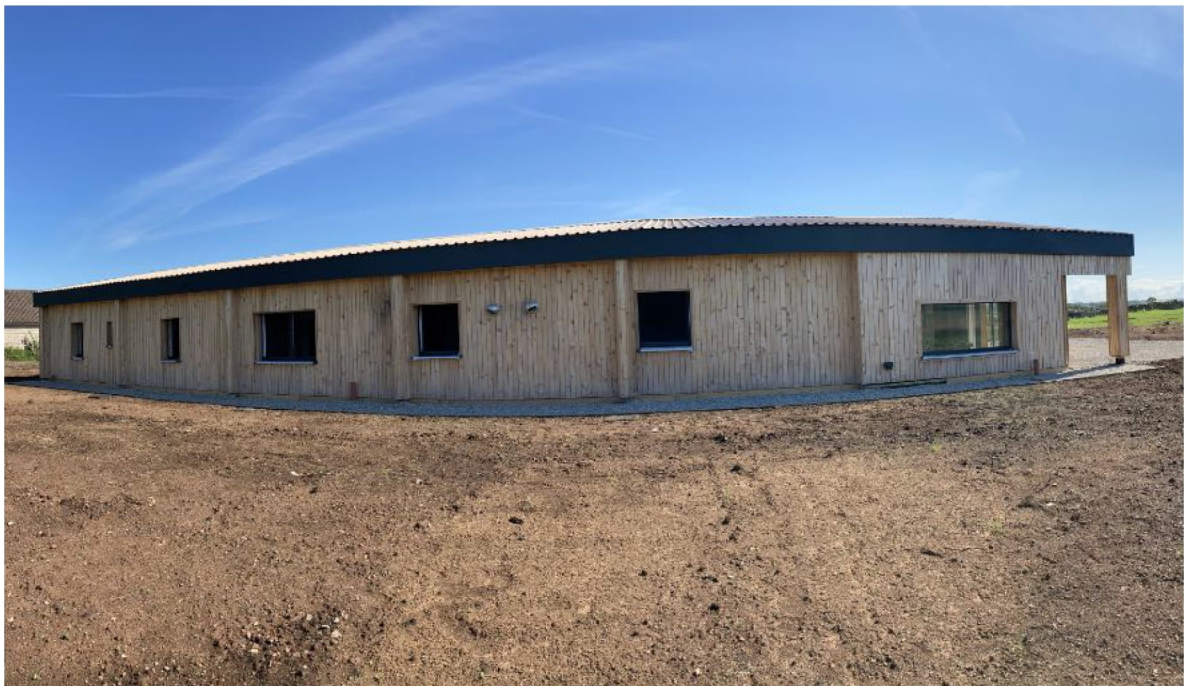
North side of the Passive house in Tickenham showing the bedroom windows and the picture window to the living room. The MVHR intake and extracts are visible in the centre.
