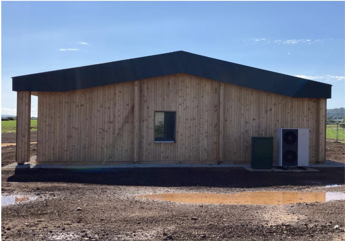
East side of the Passive house in Tickenham showing the single window to the Snug. This window provides borrowed light to the central corridor. The Air Source Heat Pump is visible on the right.
