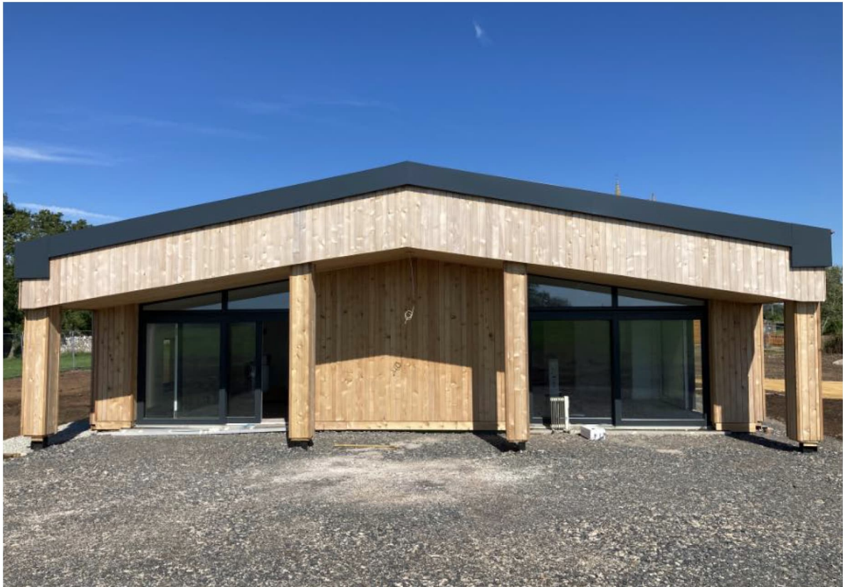
West side of the Passive house in Tickenham showing the overhanging roof that provides solar shading to the kitchen / dining / living room.
