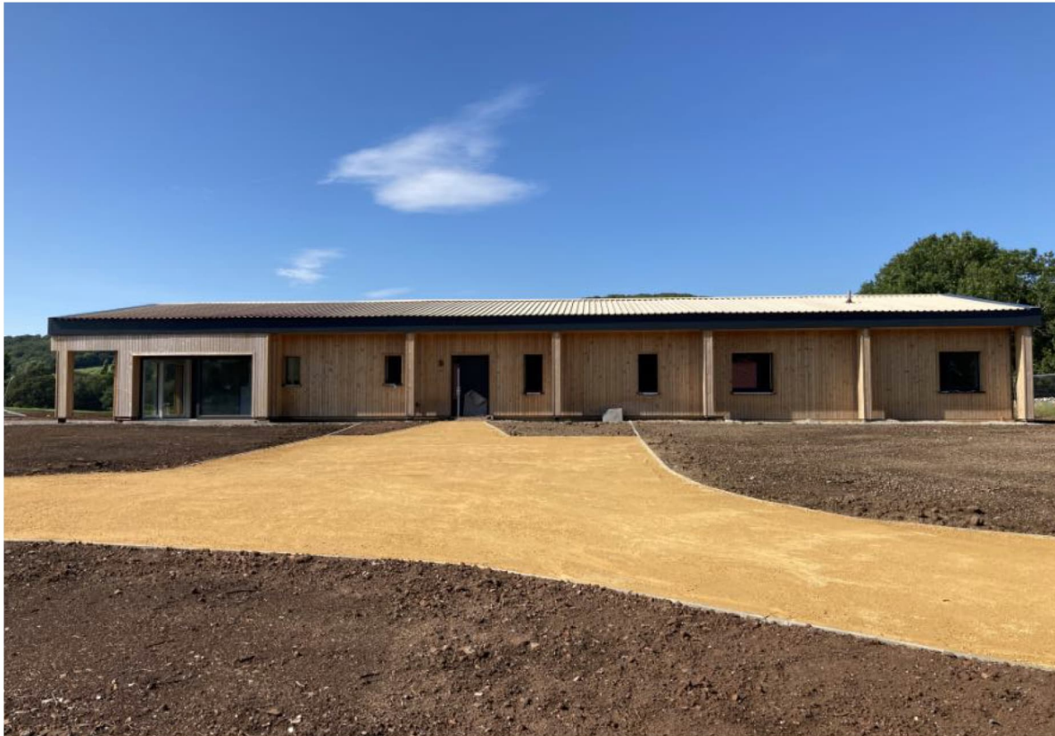
South side of the Passive house in Tickenham, a single family home. Showing the overhanging roof that provides solar shading.
