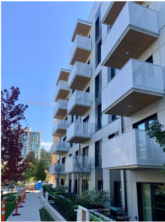
North Building Face
