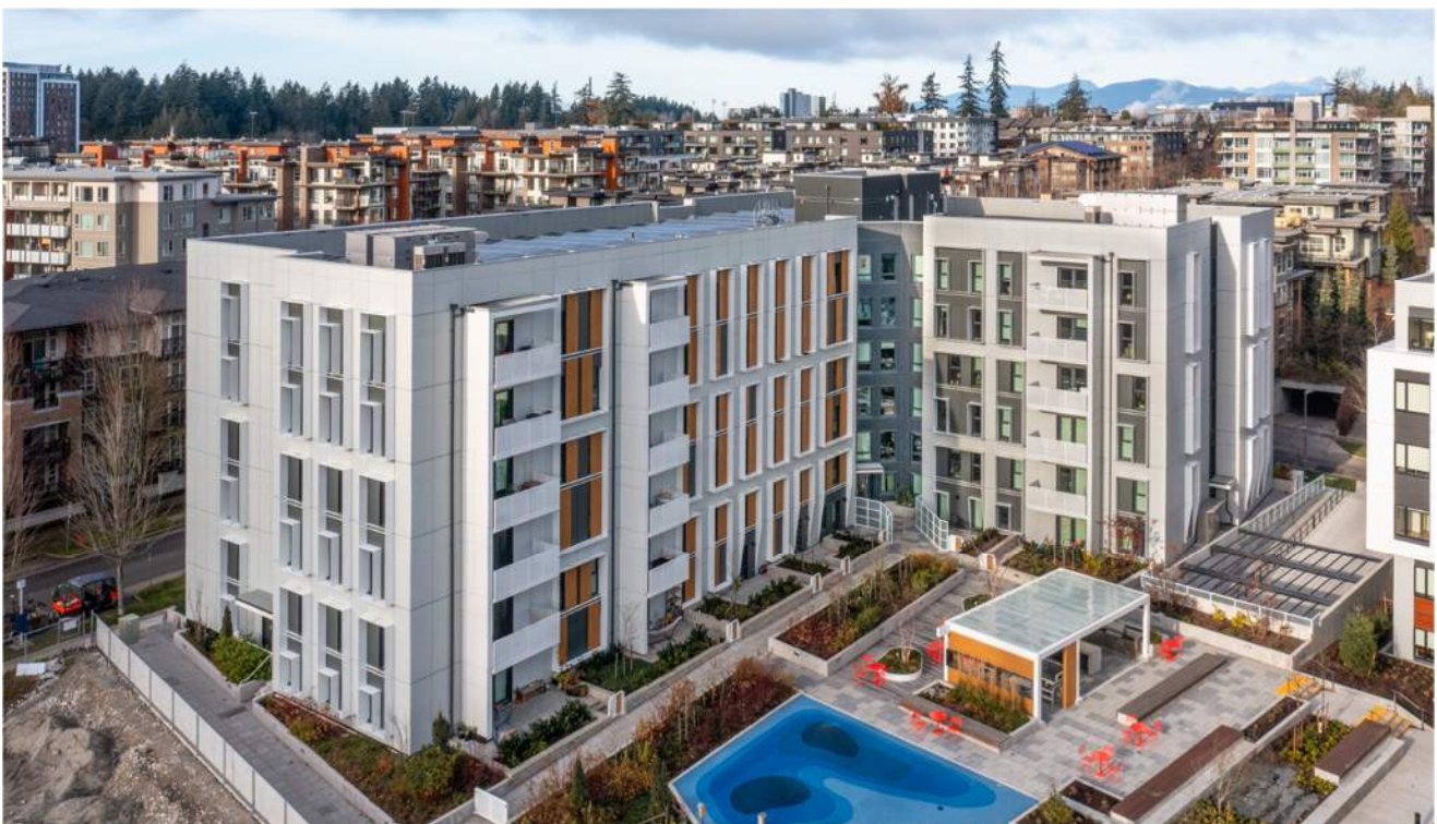
Rear of Building (East and South face of building)
