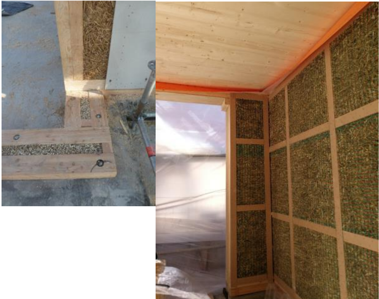
Details: Perimeter walls in wood and straw
