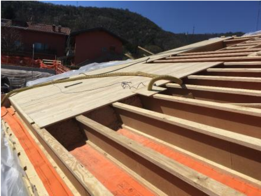
High roof: thin beam structure
