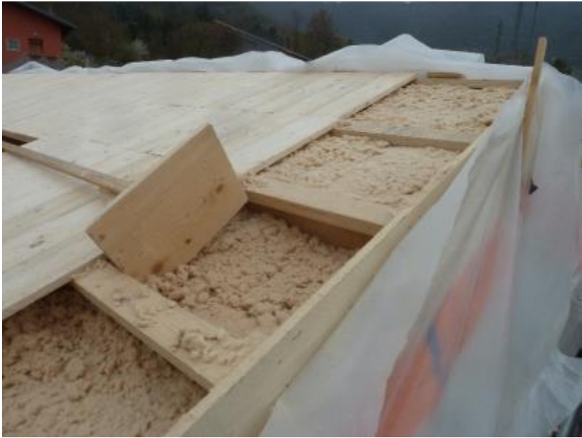
High roof: blowing phase with wood fiber
