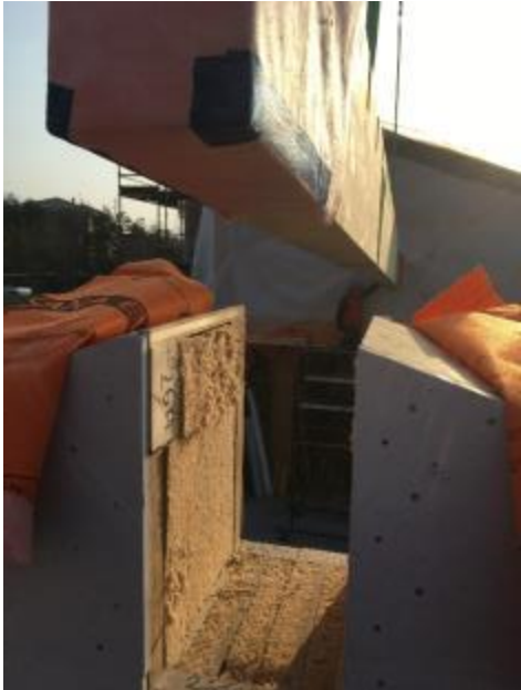
Low roof: ridge beam insulation
