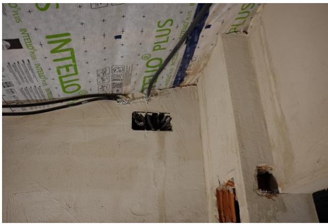
Floor and wall airtightness
