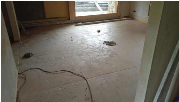
Basement floor insulation
