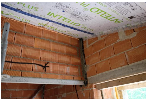
Roof airtightness
