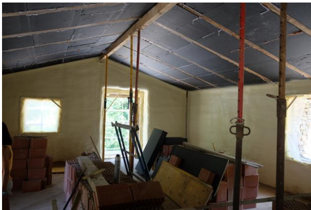
Wall and roof insulation
