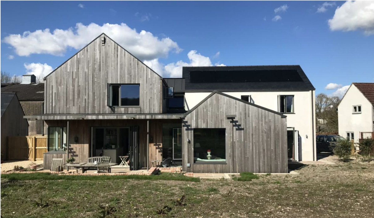
South side of the Passivhaus in Crouchestron, Wiltshire: South-facing windows are shaded by fixed horizontal overhangs to balance winter and summer solar gain. The roof mounted PV is also shown.
