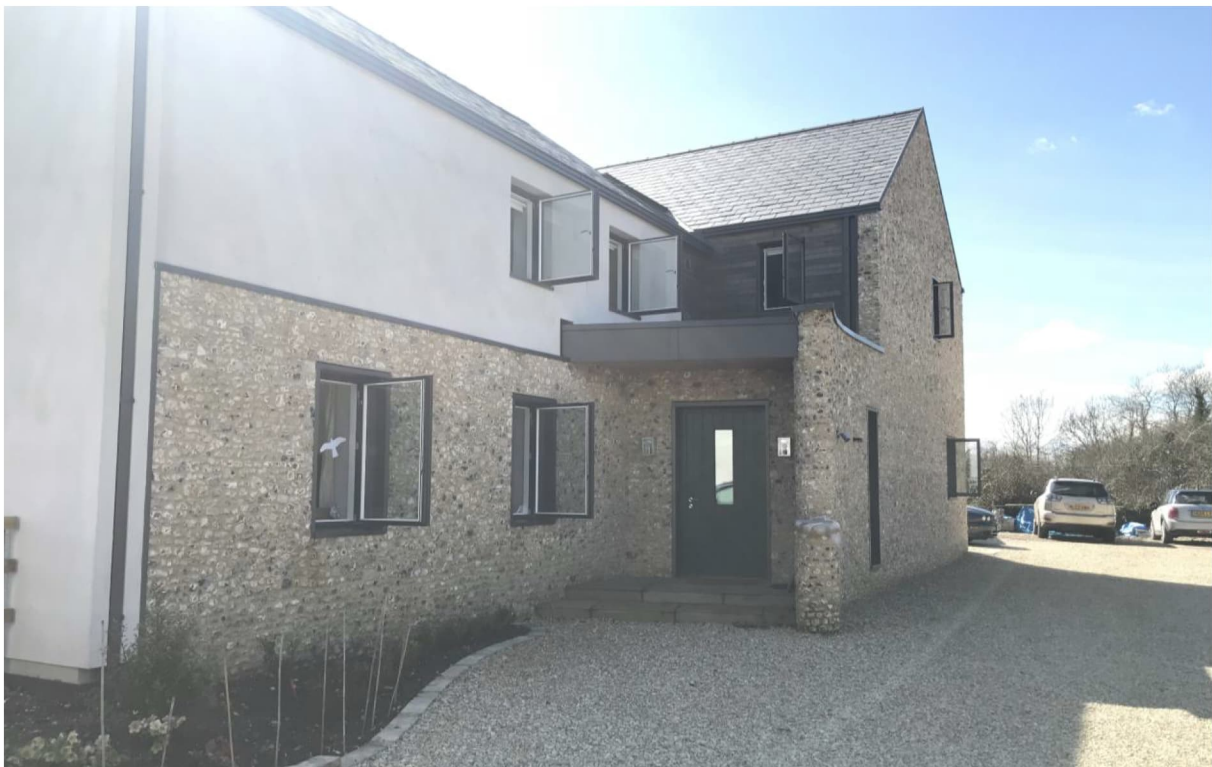
East side of the Passivhaus in Bishopstone, Wiltshire: Outward opening windows for summer comfort ventilation can clearly be seen.
