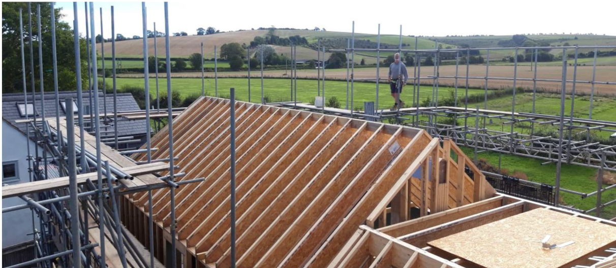
Fig. 5: Timber frame roof in construction.
