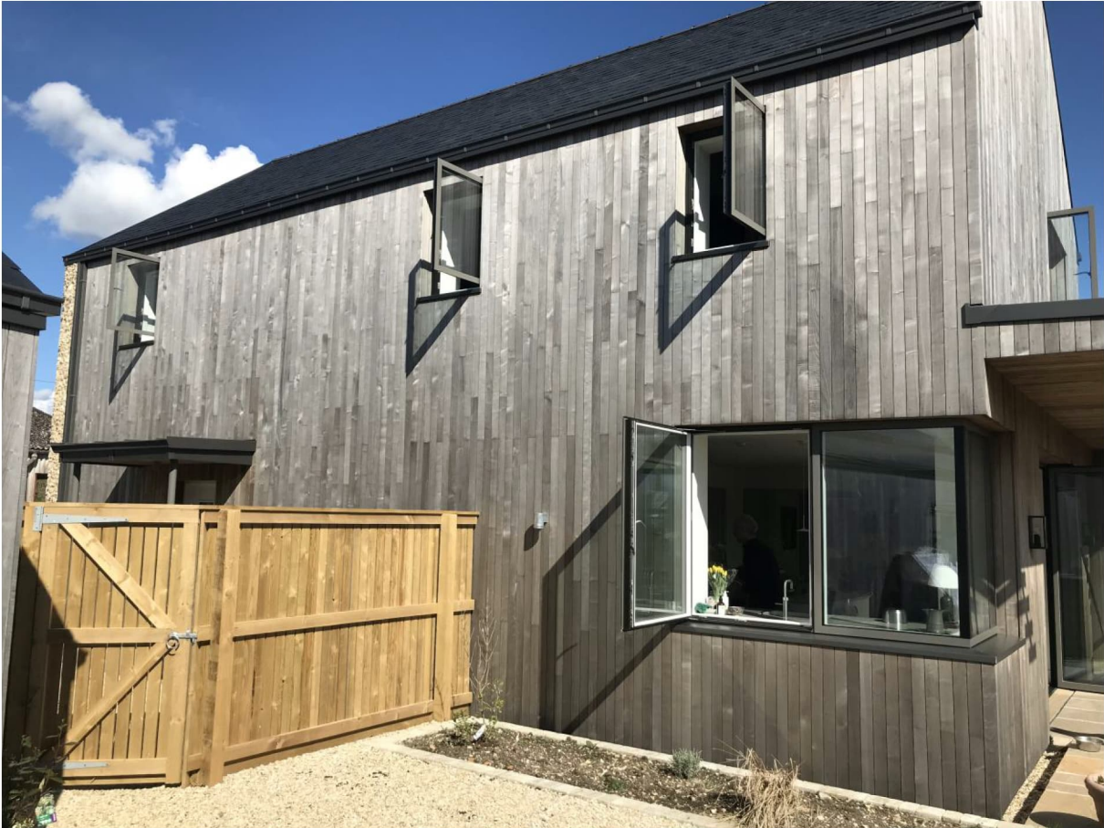
West side of the Passivhaus in Bishopstone, Wiltshire: Outward opening windows for summer comfort ventilation and the utility room porch canopy are shown.
