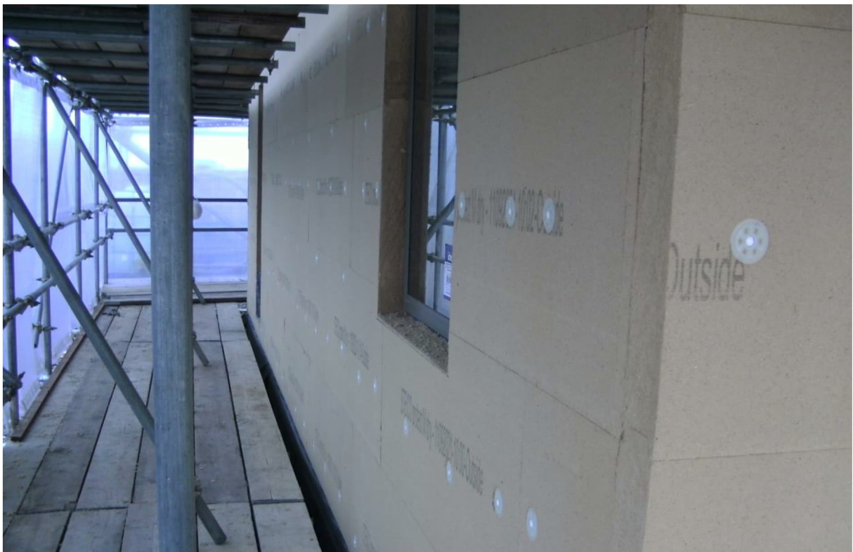
Fig. 4: Rigid woodfibre board applied externally before installation of rainscreen.
