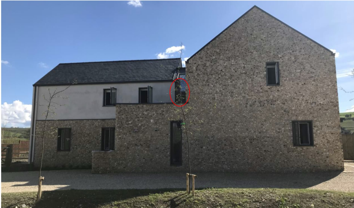
North side of the Passivhaus in Bishopstone, Wiltshire: MVHR ventilation grilles are just visible (circled red).
