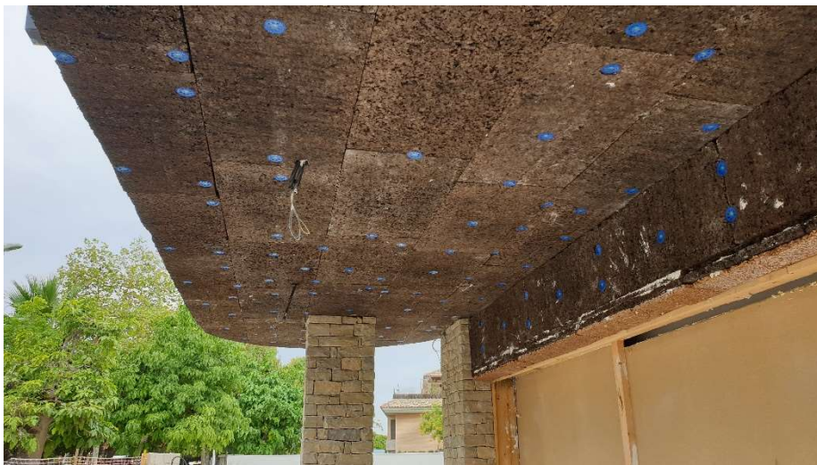
ETICS installation (Source: Amalur Arquitectura)
