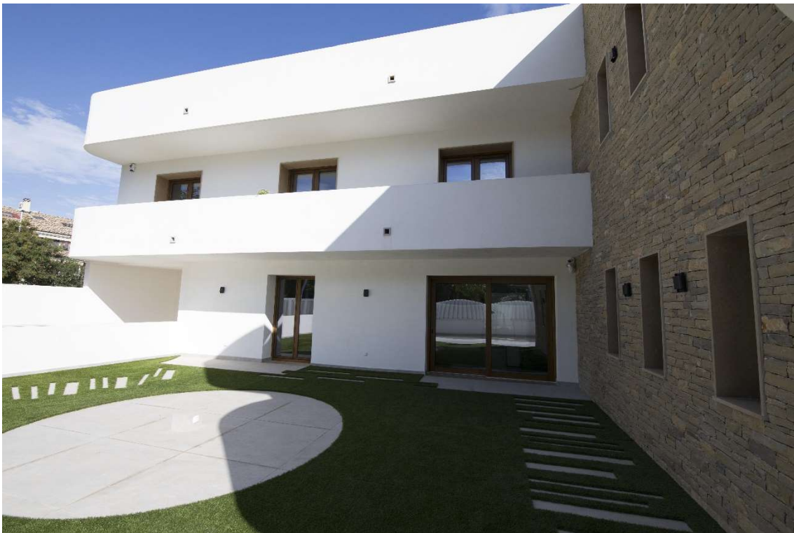
South view - (Source: Amalur Arquitectura)
