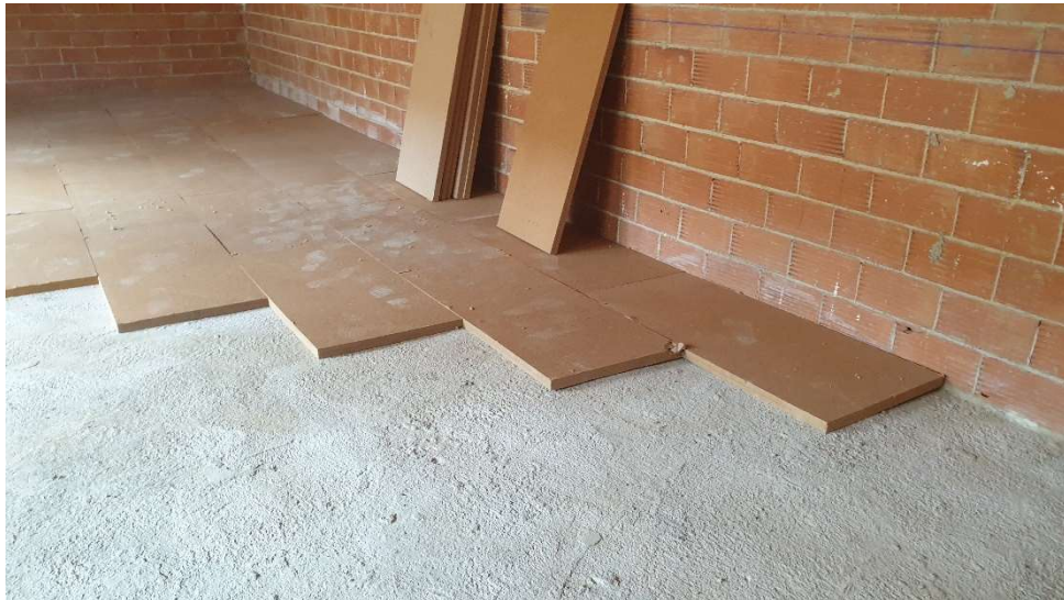
Basement floor insulation (Source: Amalur Arquitectura)
