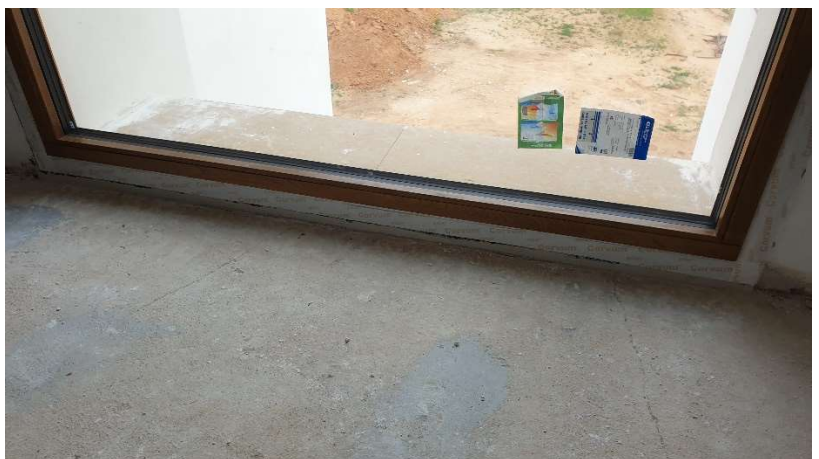
Window installation (Source: Amalur Arquitectura)
