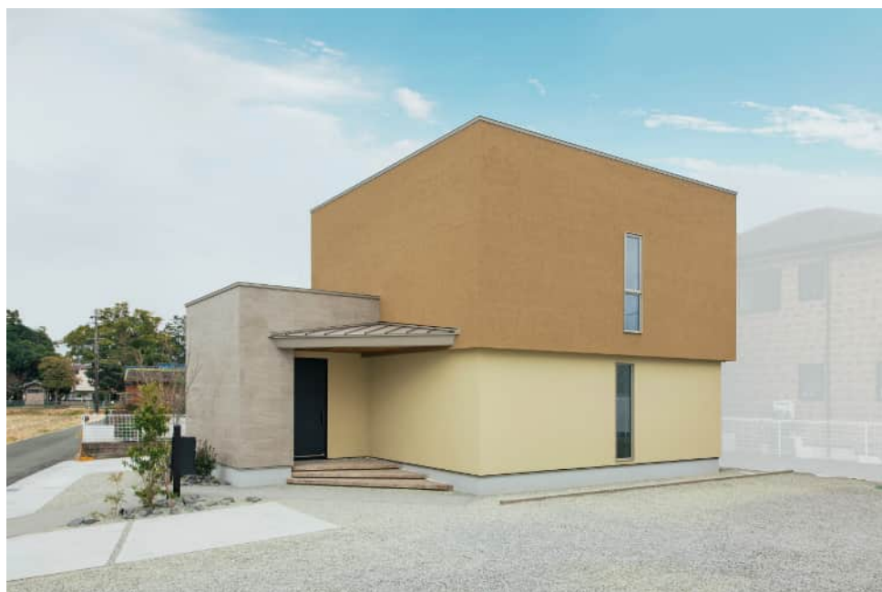
View from Southwest
