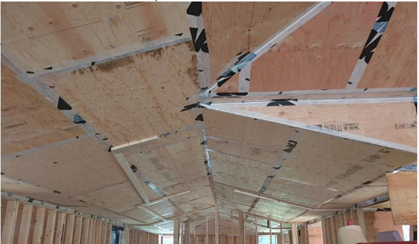
Plywood sheathing, tape sealing photographed during construction.
