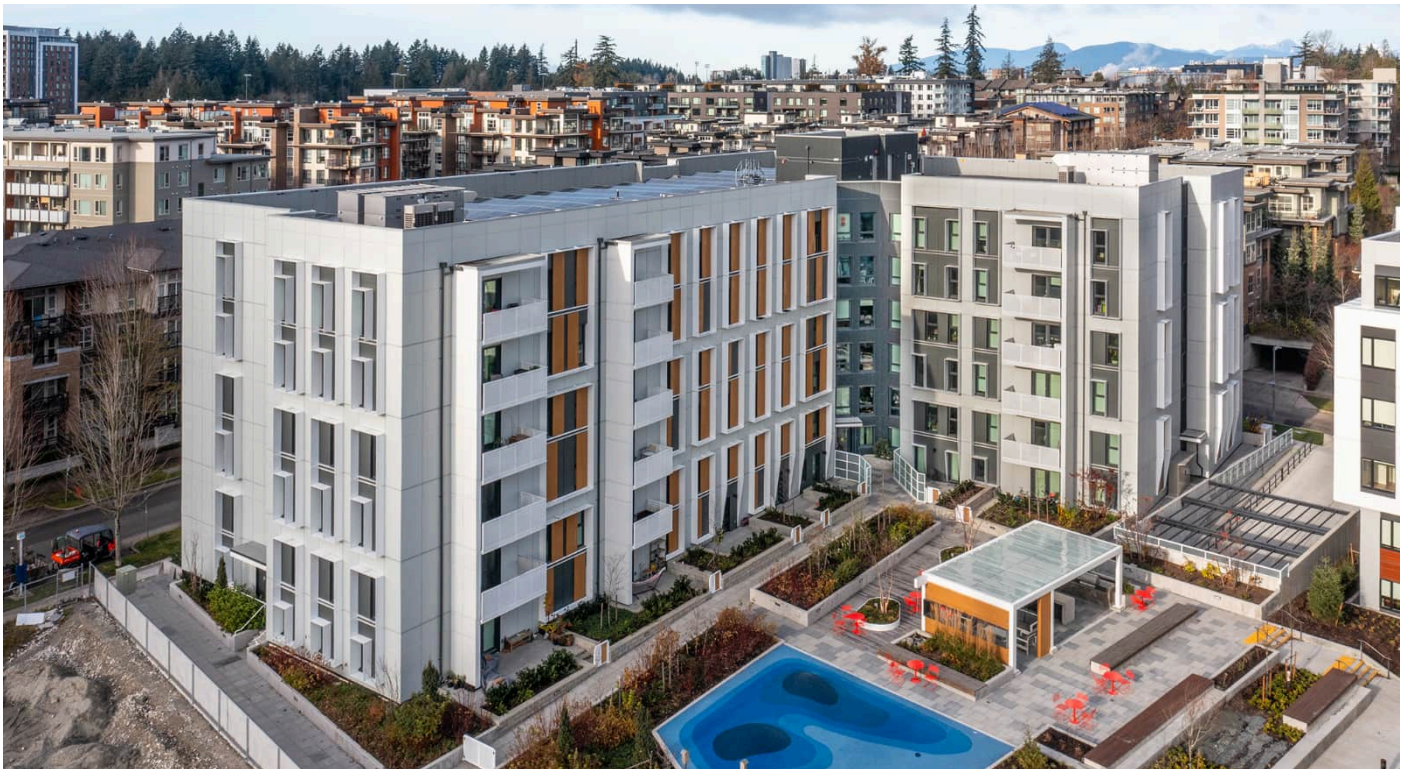
Rear of Building (East and South face of building)
