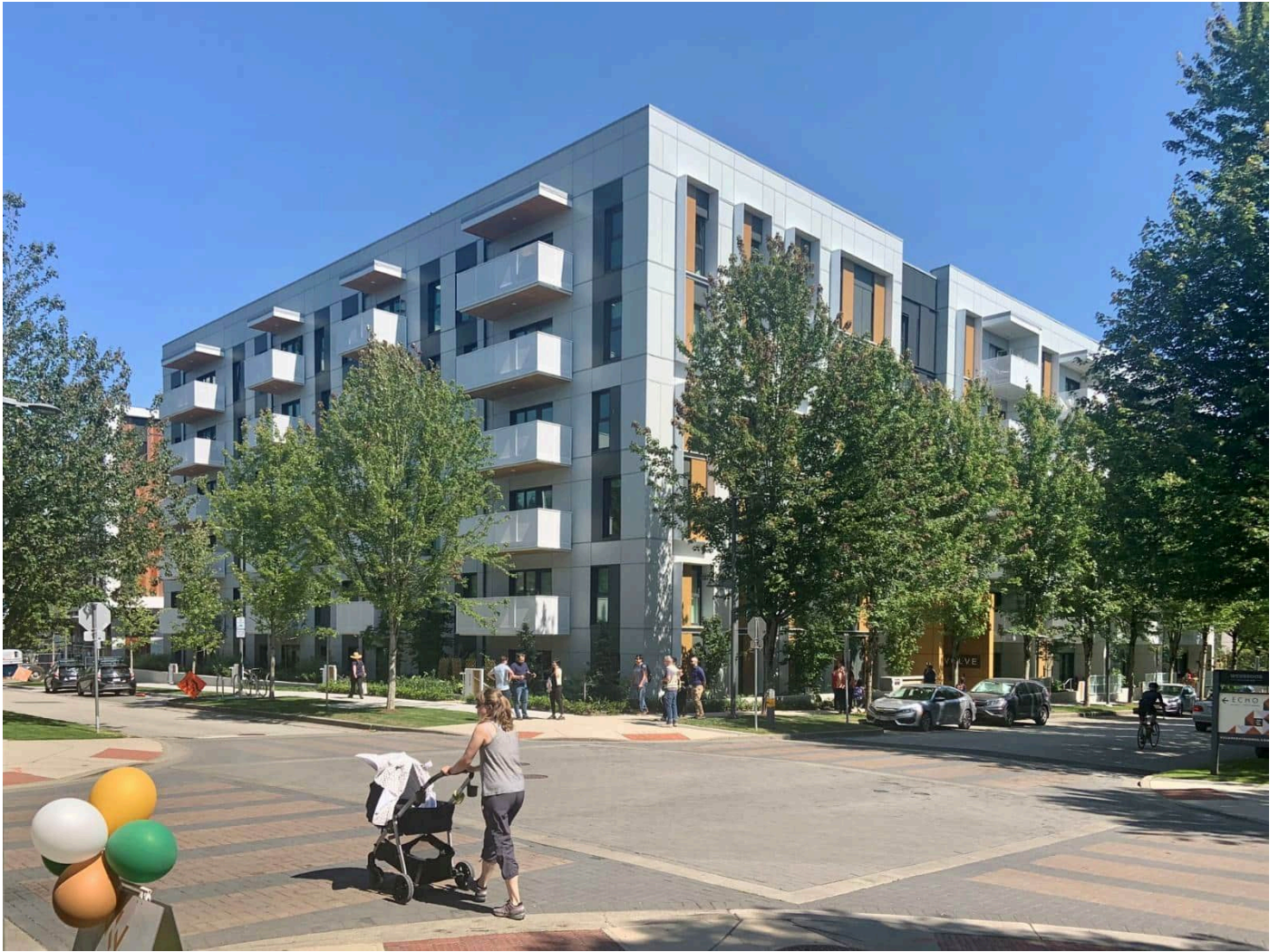
North-West Corner of Building
