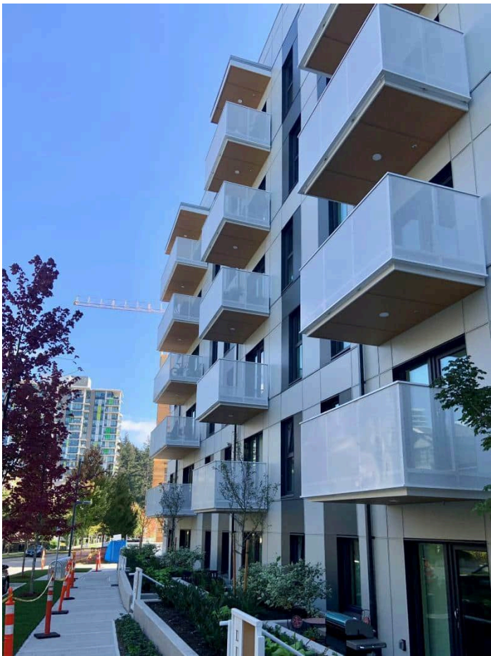
North Building Face
