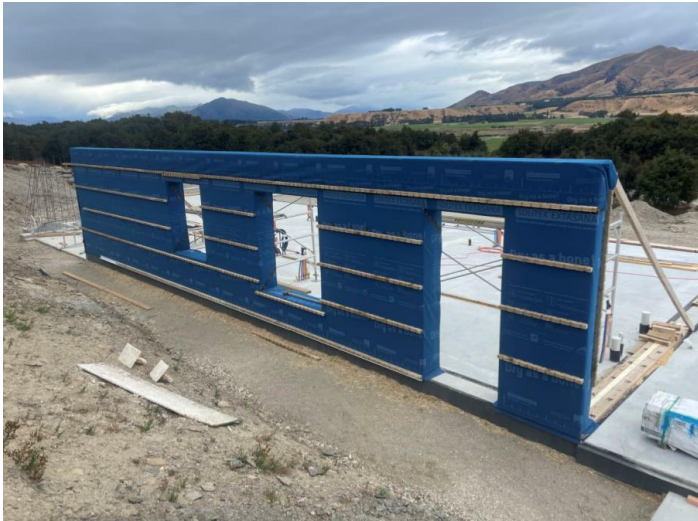
Exterior airtight membrane on straw panel walls and concrete slab
