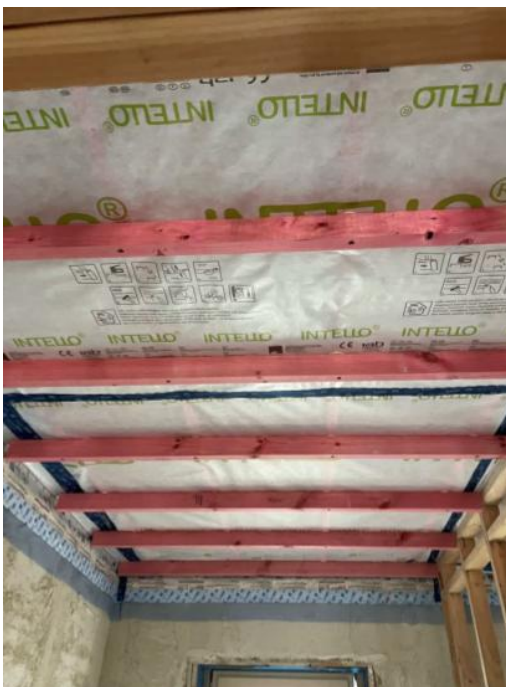
Internal airtight membrane to roof and wall corner
