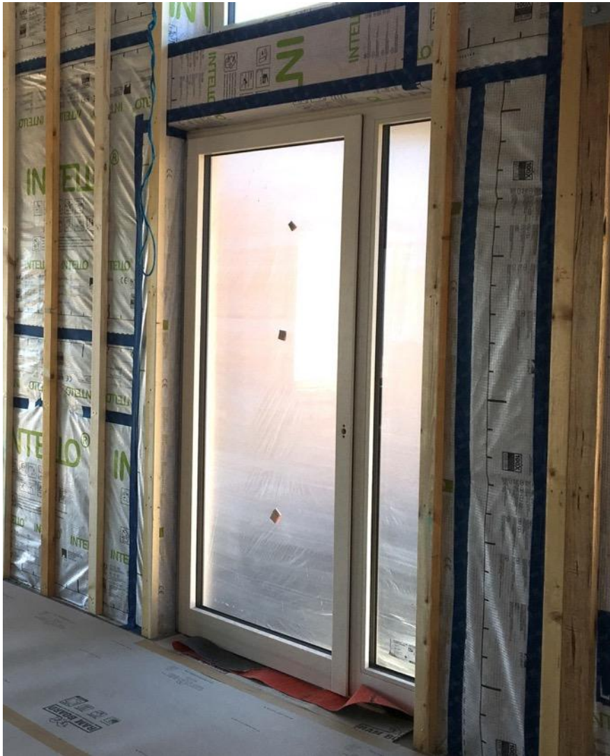
Windows – interior view
