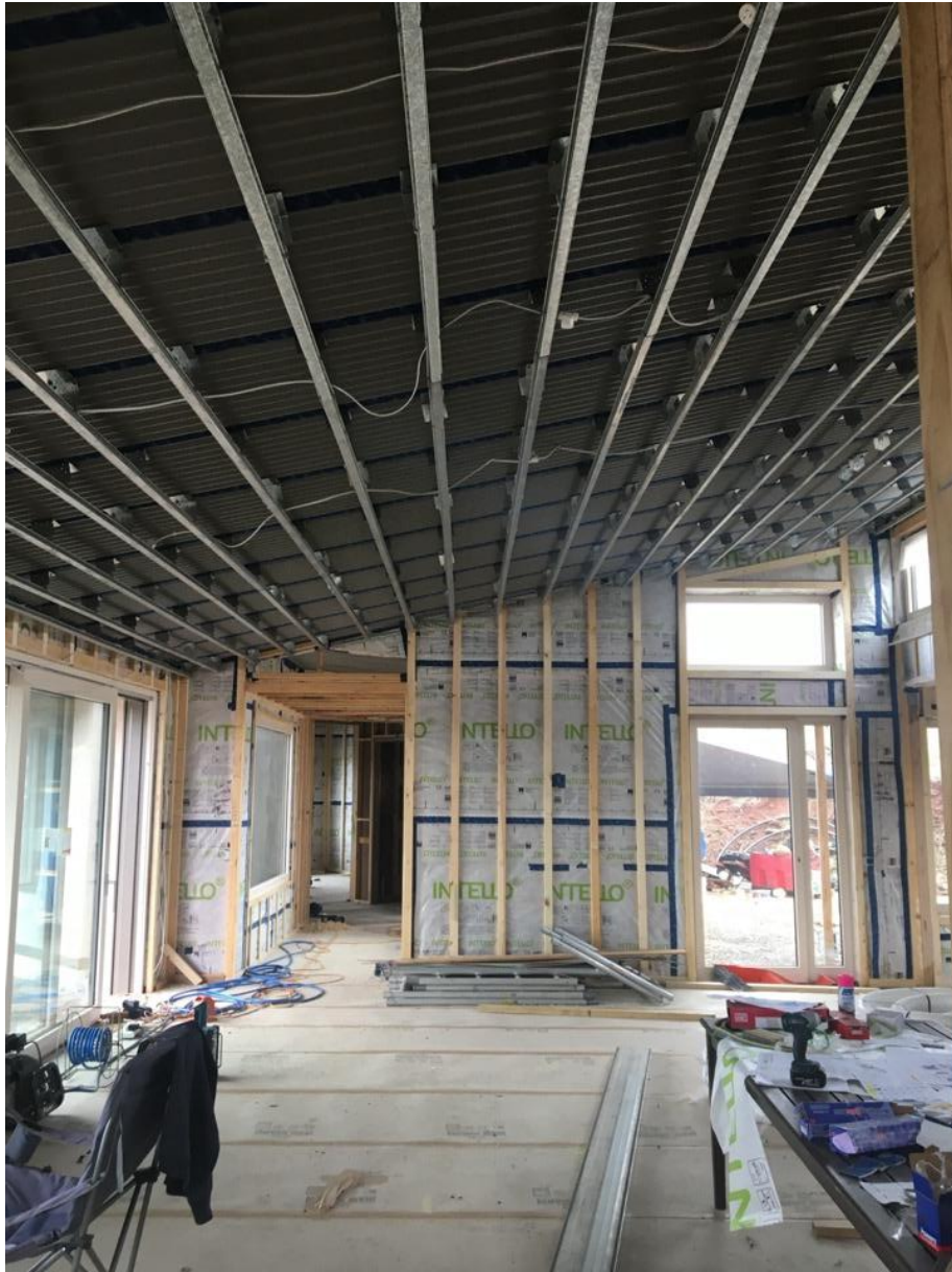
Interior airtightness membranes
