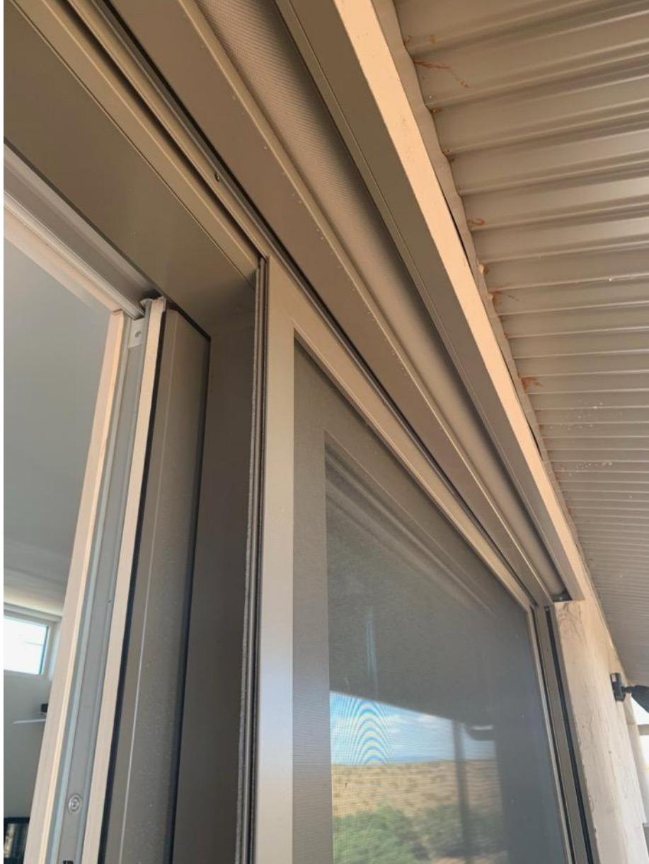
Windows – exterior view
