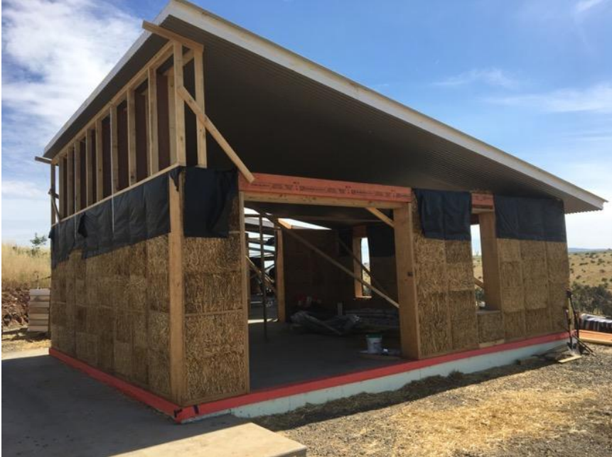
Roof during construction
