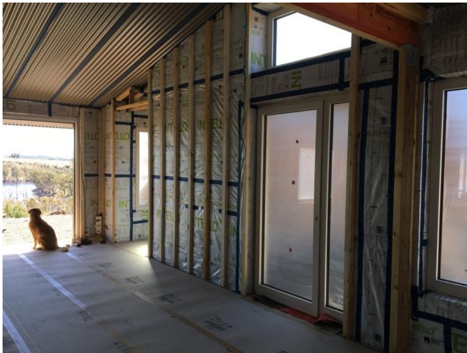
Walls during construction – internal view
