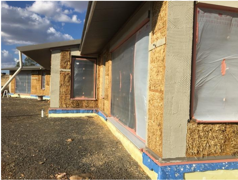
Walls during construction – external view
