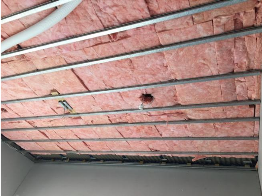
Roof interior side insulation
