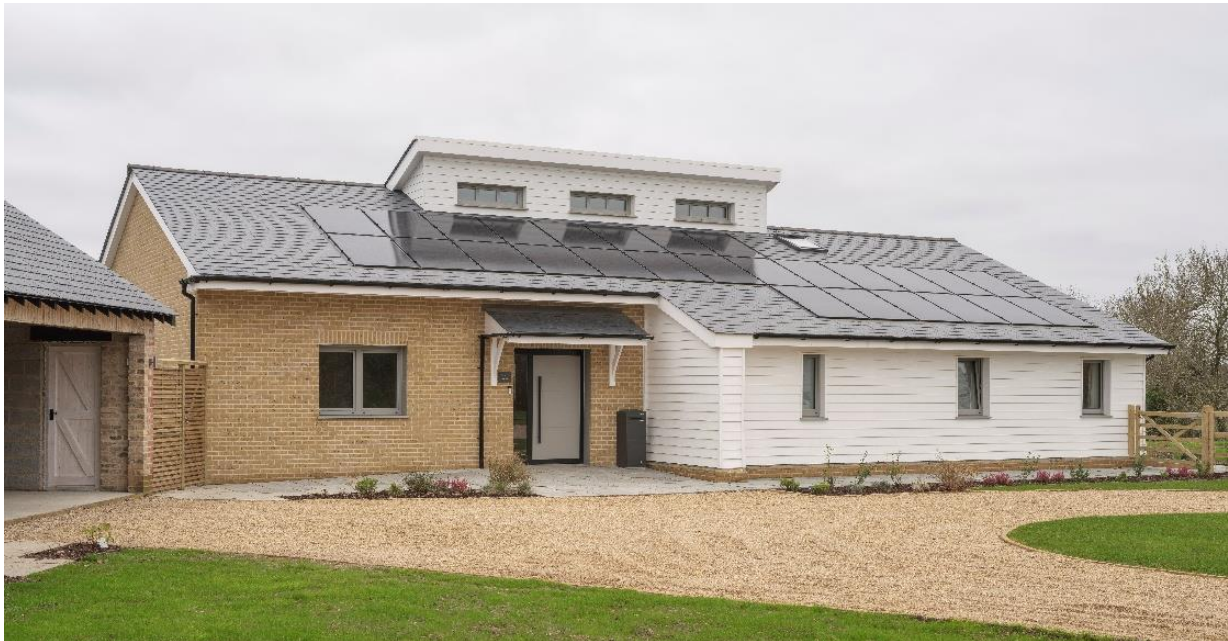
Avery Lodge, detached single storey bungalow with mezzanine. Sacombe Green, Farm, Ware SG12 0JF
