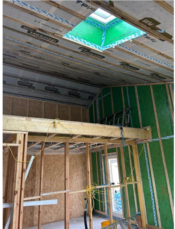
Purge and night time ventilation through rooflights and clearstory window.
