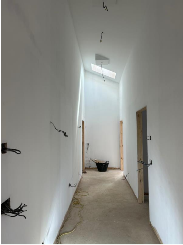
Purge and night time ventilation through rooflights and clearstory window.
