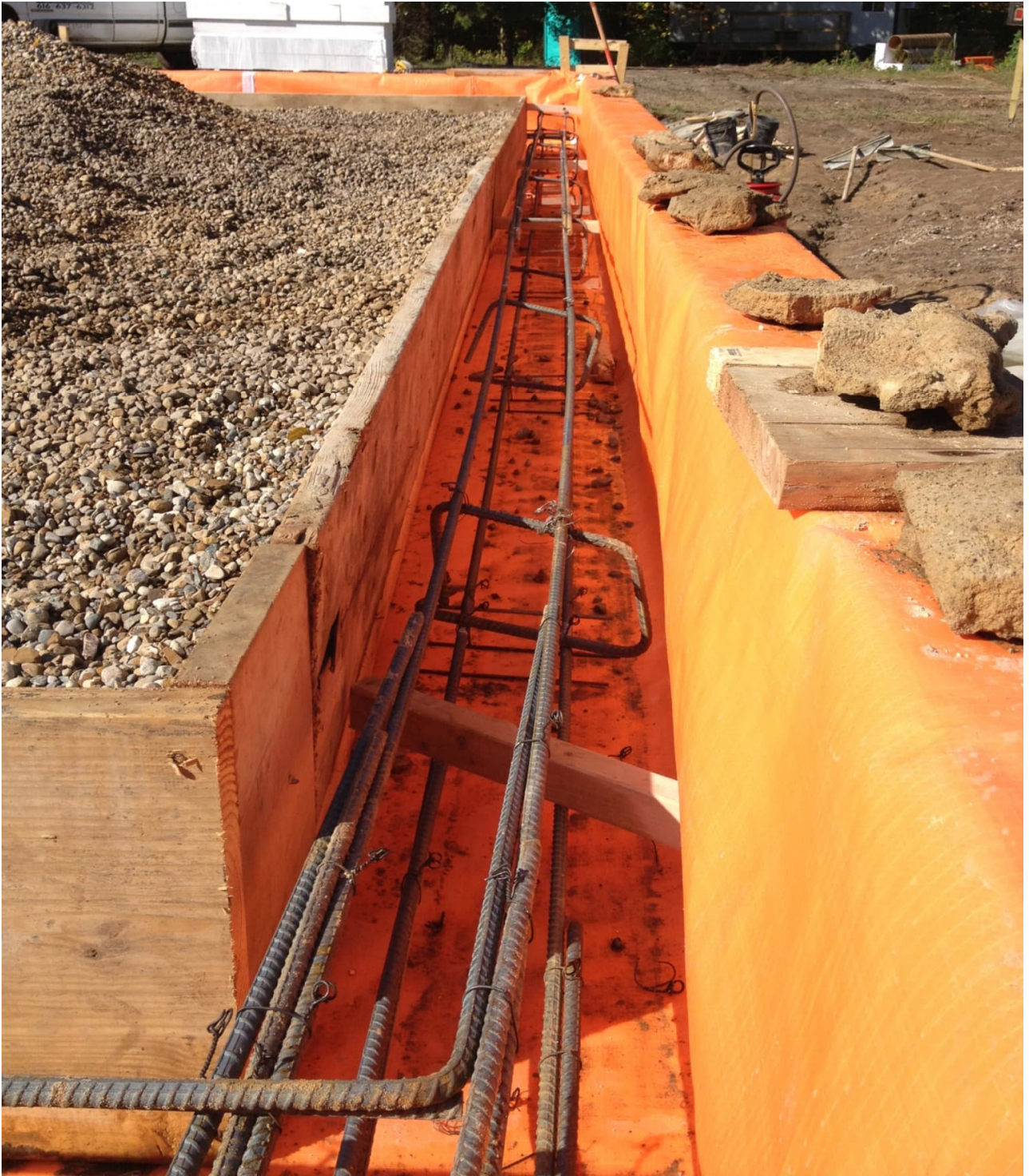
Underslab air barrier at foundation edge
