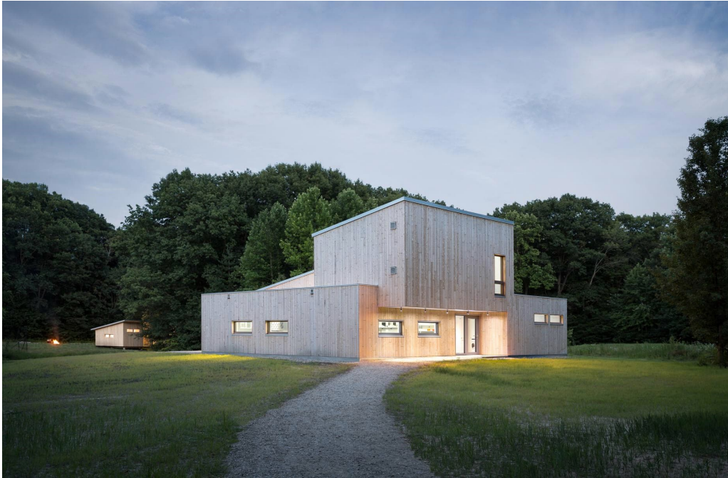
View from the Northwest
