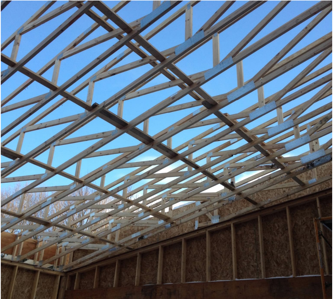
Roof truss installation
