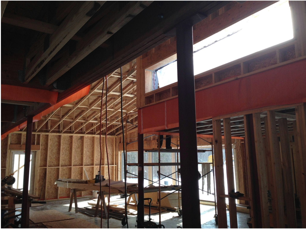
View of pre-installed flexible air barrier transitions during framing
