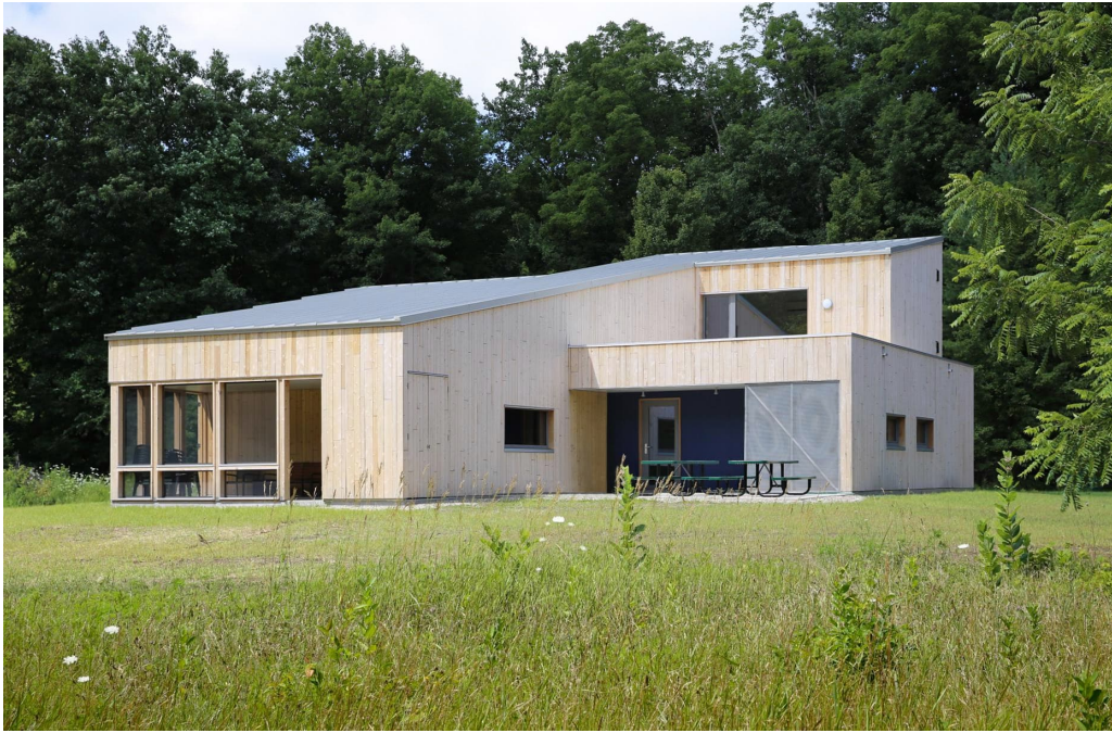
View from the Northeast
