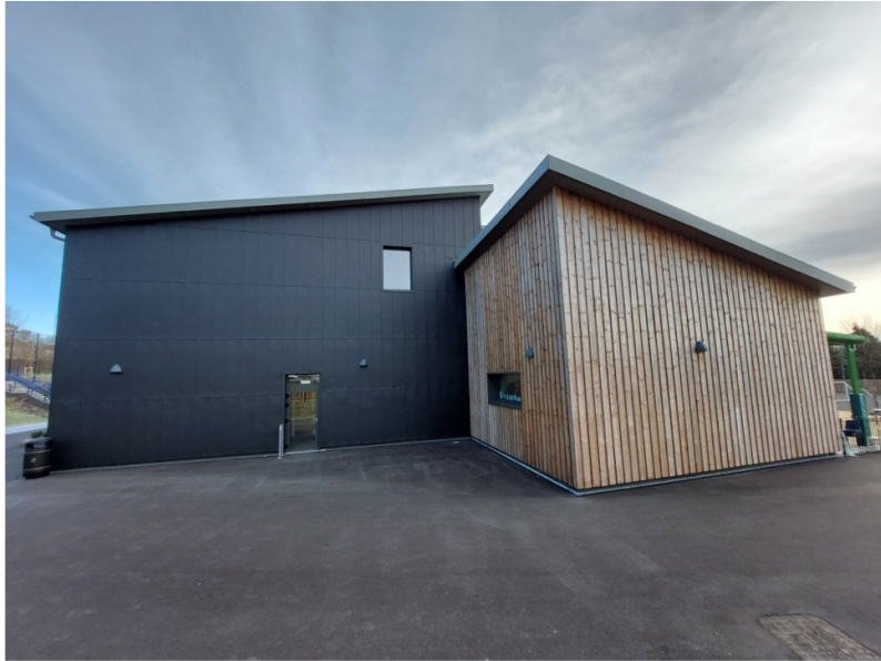
Gorslas Primary School, View from west
