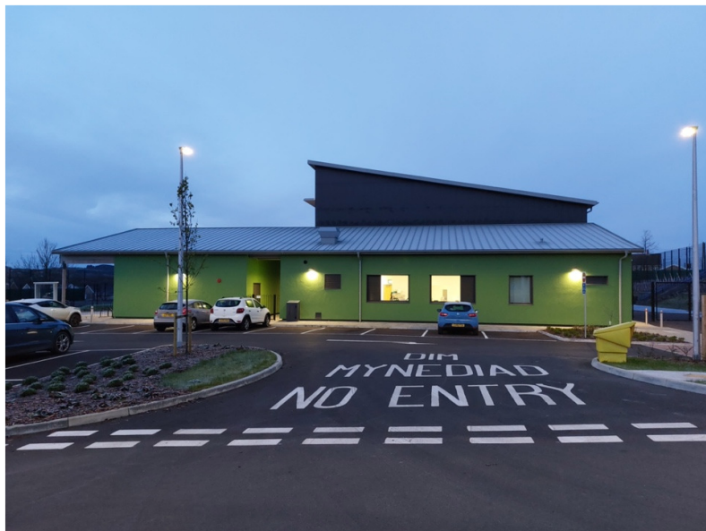
Gorslas Primary School, View from east
