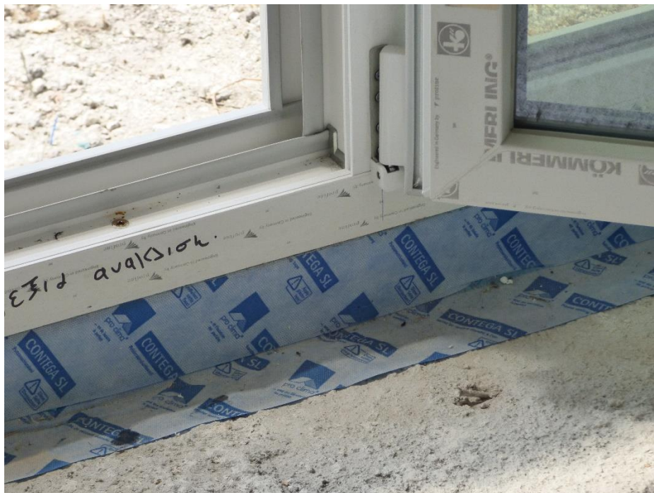
Picture 23: Windows installation
