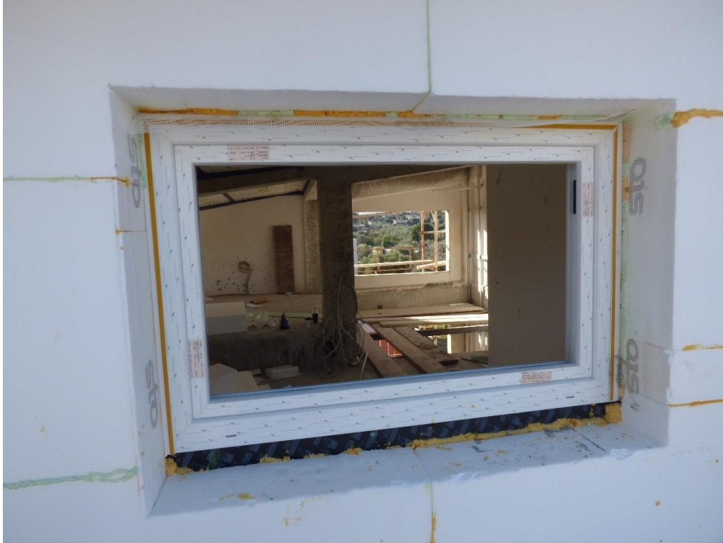
Picture 20: Window installation
