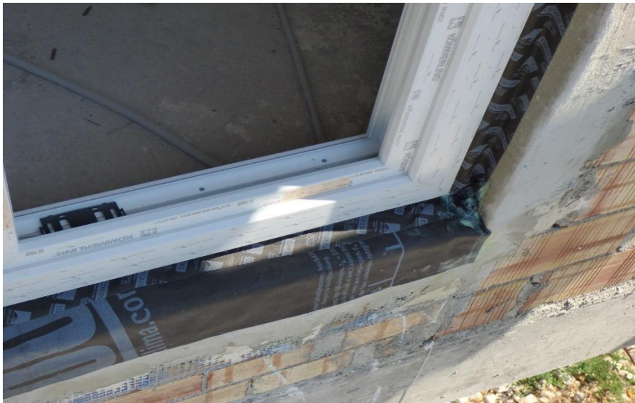
Picture 22: Windows installation
