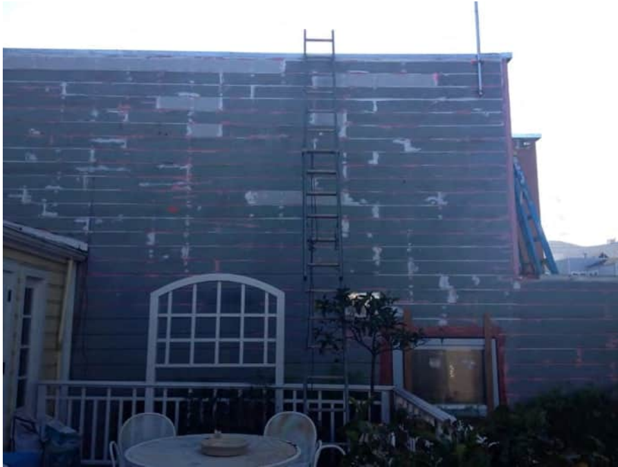
Side, East (In Progress)
