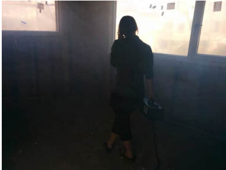
Smoke Testing the Envelope for Leaks
