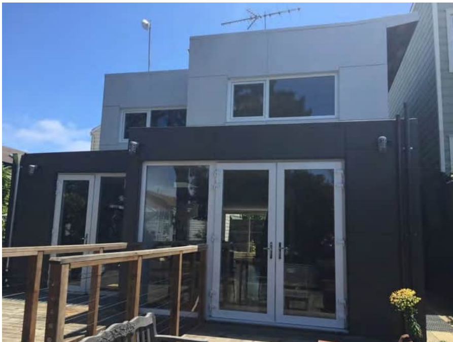
Rear, North (After)
