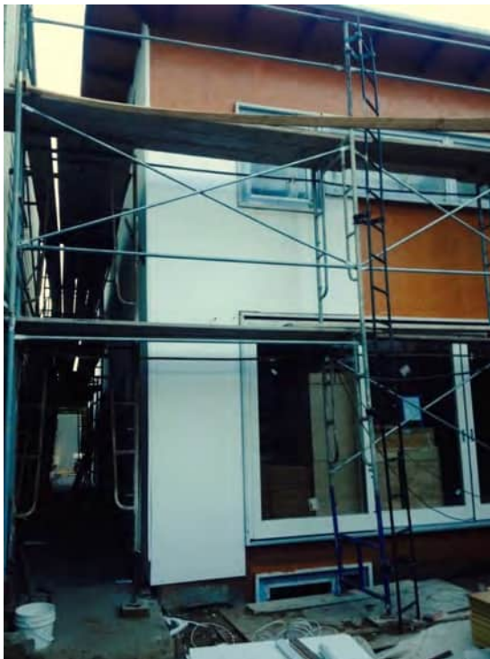
Photo of Exterior of South Wall, EPS Insulation Being Installed
