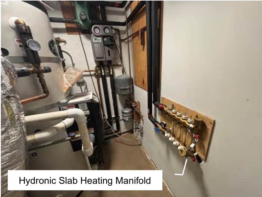
Distribution Manifold for Hydronic Slab Heating, Right Foreground
