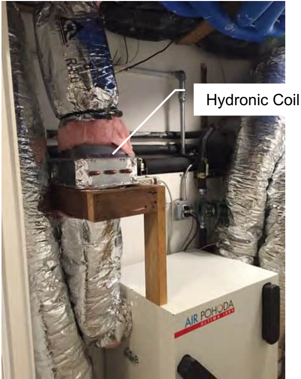
Hydronic Heating Coil in Ventilation Air Supply
