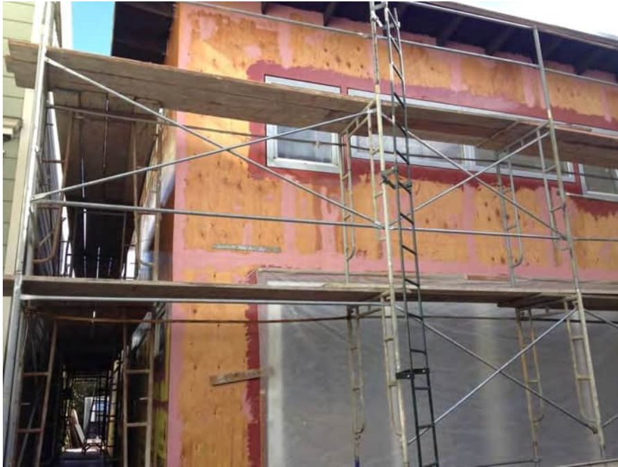
Photo of Exterior of South Wall
