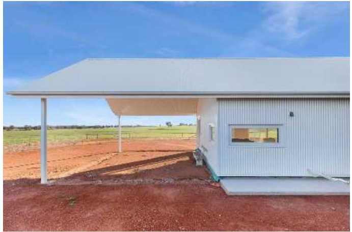
Southern elevation showing alfresco and living room window
