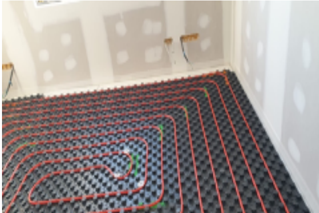
Radiant floor installed
