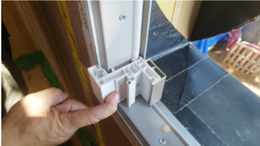
Demonstration of fit Casement frame with Mounting frame
