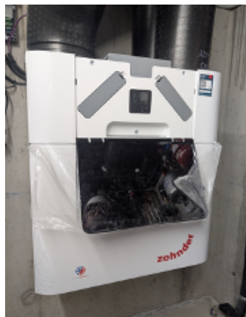
Zehnder ComfoAir Q600 Photo ZEST architecture
