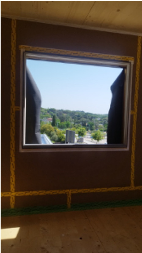
View of 3 types of Siga seal band installed
