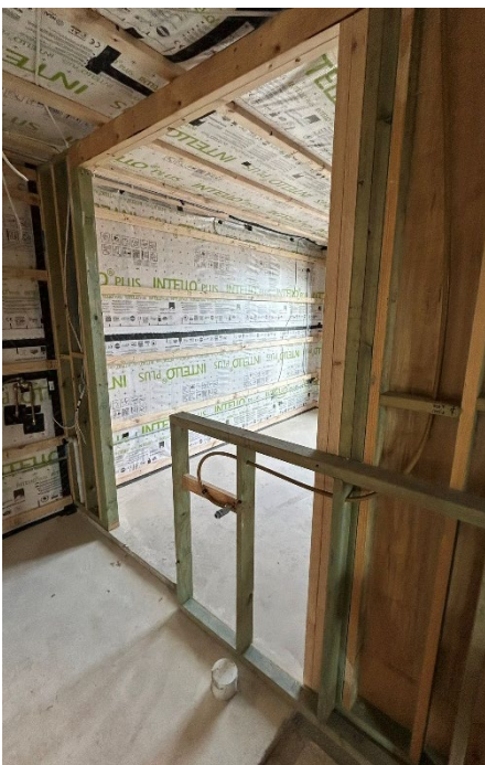
Construction shot - Internal view
