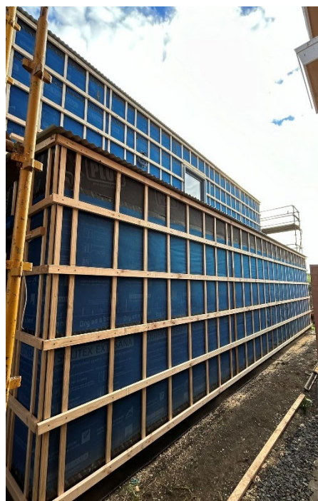
Construction shot - external view
