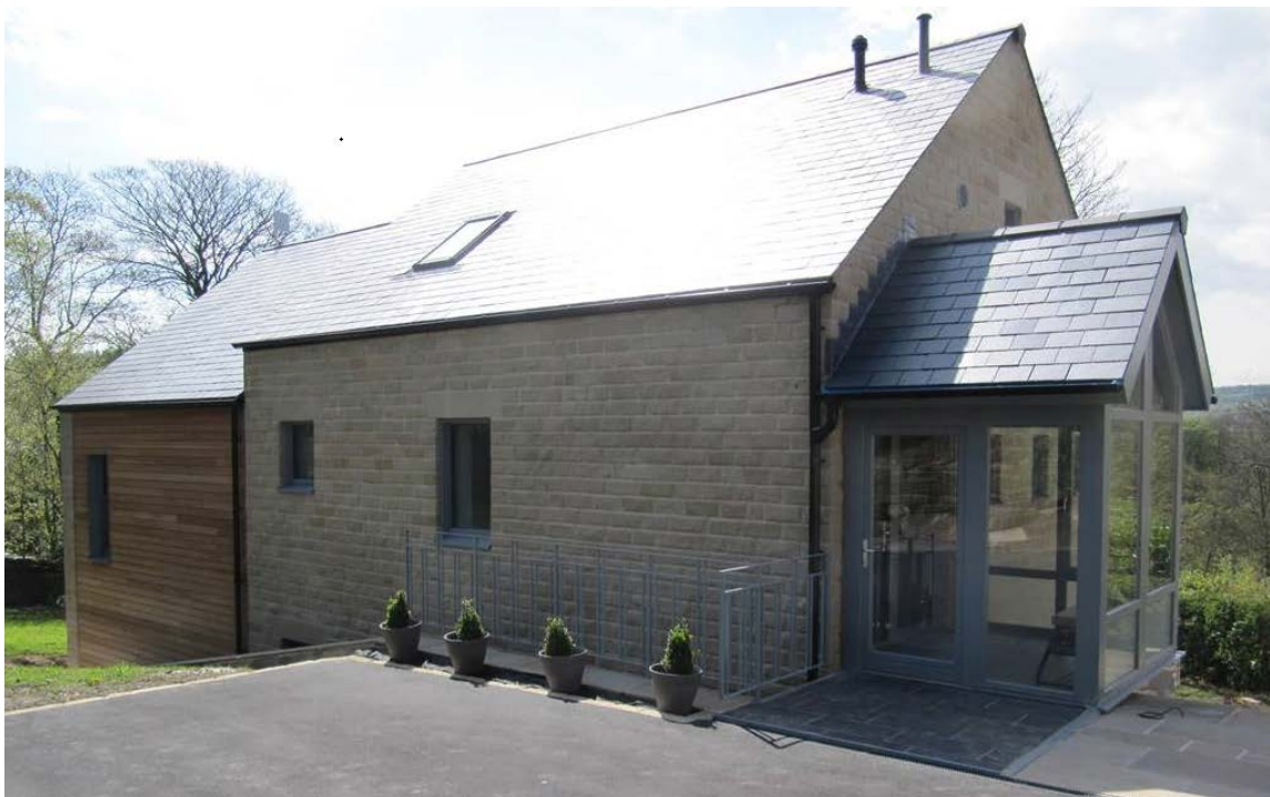
Picture of the Passive House in Huddersfield West Yorkshire from the north ; entrance lobby to the first floor living areas and optimised glazing areas can be seen.
