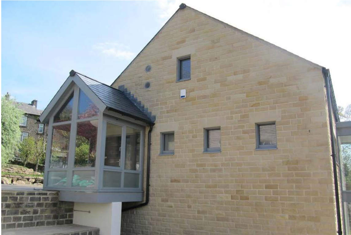
West side of the Passive House in Huddersfield, West Yorkshire; The intake and exhaust air grilles for the MVHR system are clearly visible, this elevation faces a public road, the windows were sized for adequate daylighting.
