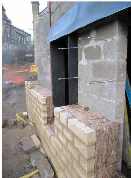
Fig 3. Full fill cavity insulation and basalt wall ties.
