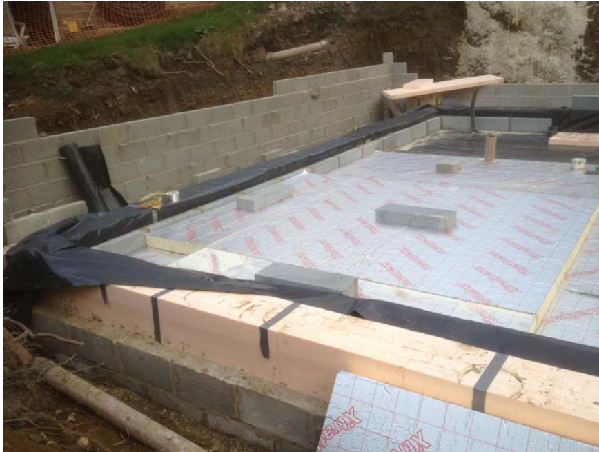
Fig 1. Slab and perimeter insulation, installation.
