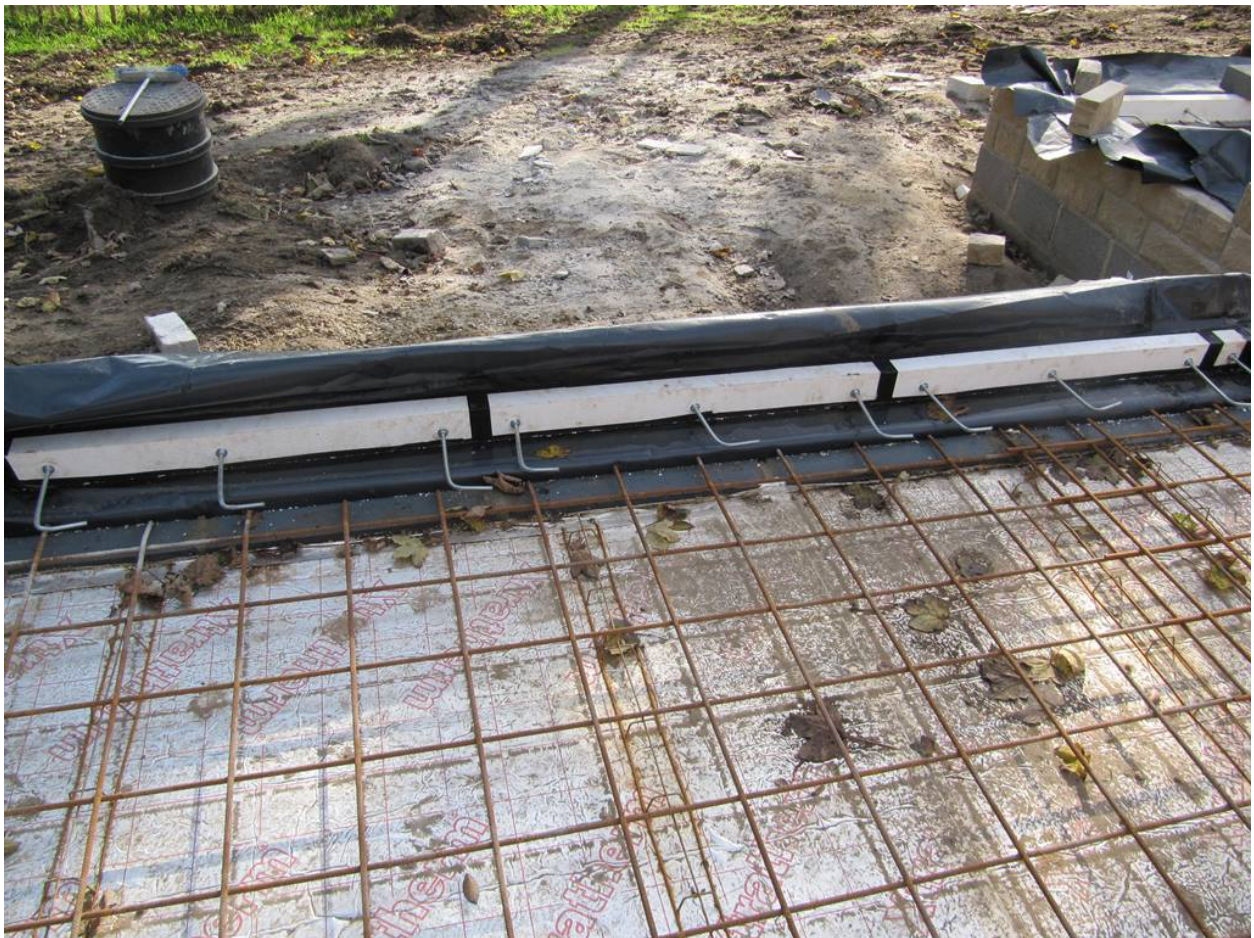
Fig 2. Compacfoam positioned to be cast into slab to reduce thermal bridge at thresholds.
