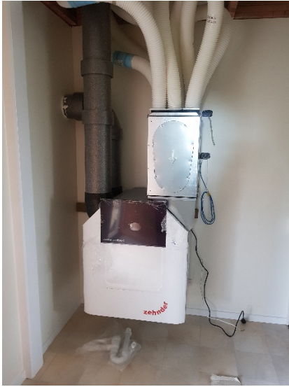
Figure 26 Zehnder ComfoAir Q350 during installation
