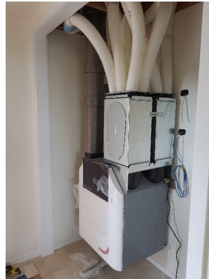
Figure 25 Zehnder ComfoWell attenuators above central unit
