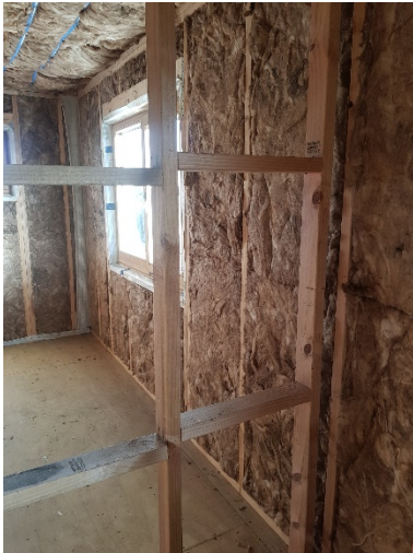
Figure 13 Insulation to the wall studs
