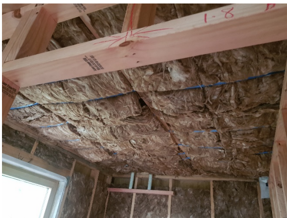
Figure 17 Roof / ceiling insulation
