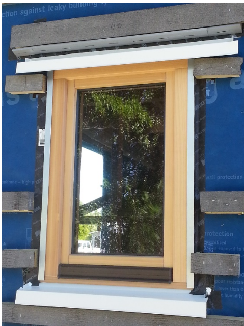
Figure 22 External view of window taped in place
