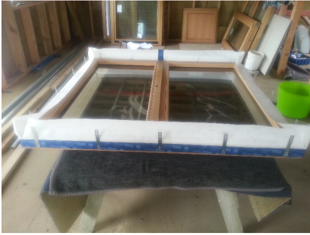
Figure 21 Window taped & fixing brackets attached
