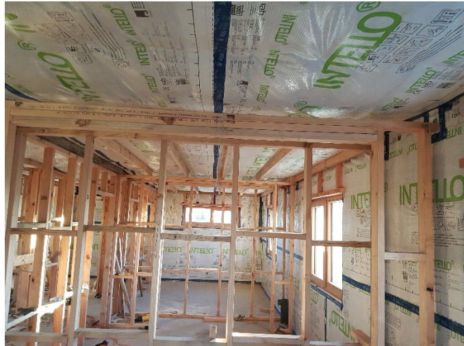
Figure 12 Typical Intello airtightness layer installed to the wall studs and first floor ceiling, with joints taped
