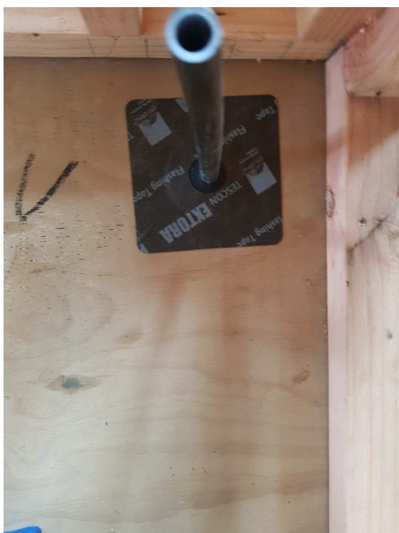
Figure 24 Typical Air Seal – Pipe to plywood floor
