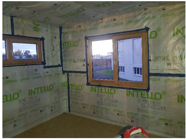
Figure 20 Window installed and taped to Intello airtight layer on wall framing
