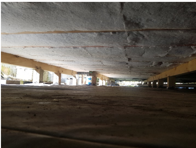
Figure 9 2 layers of Polyester underfloor sections between joists
