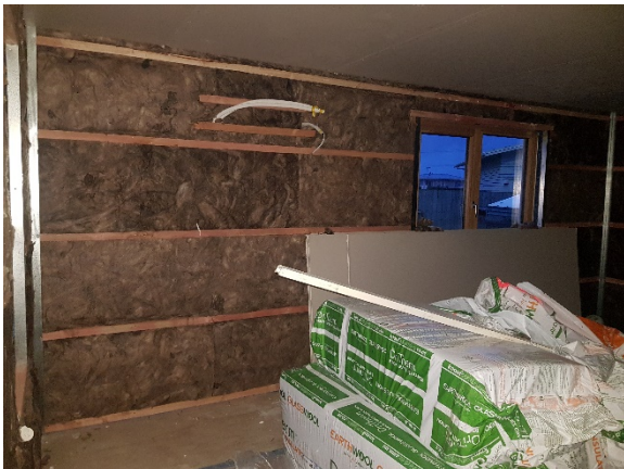
Figure 14 Insulation to the horizontal service cavity inside the airtightness layer
