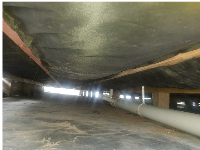
Figure 8 Additional layer of glasswool insulation with windwash, perpendicular to and under the joists
