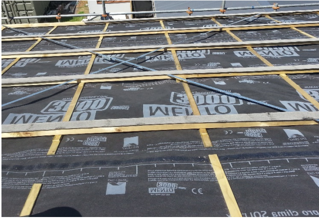
Figure 18 Roof purlins on counterbattens on roofing underlay
