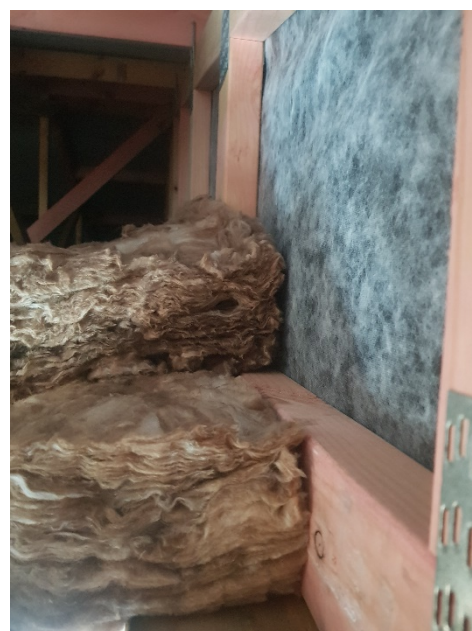
Figure 16 2 layers of insulation to roof space
