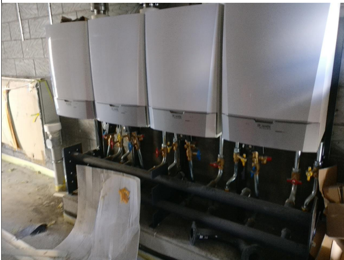
Thermally isolated pipe supports, during installation.
