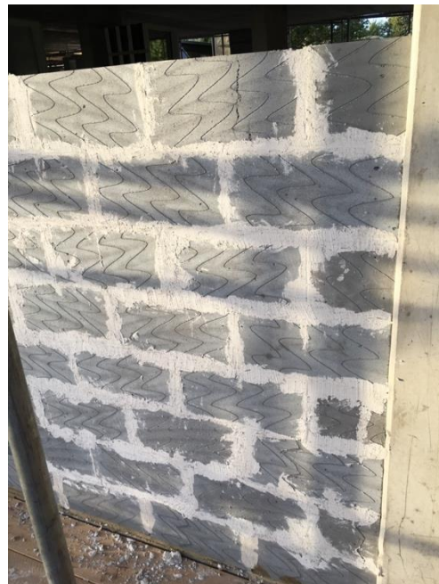
Inner leaf of AAC lightweight blockwork
