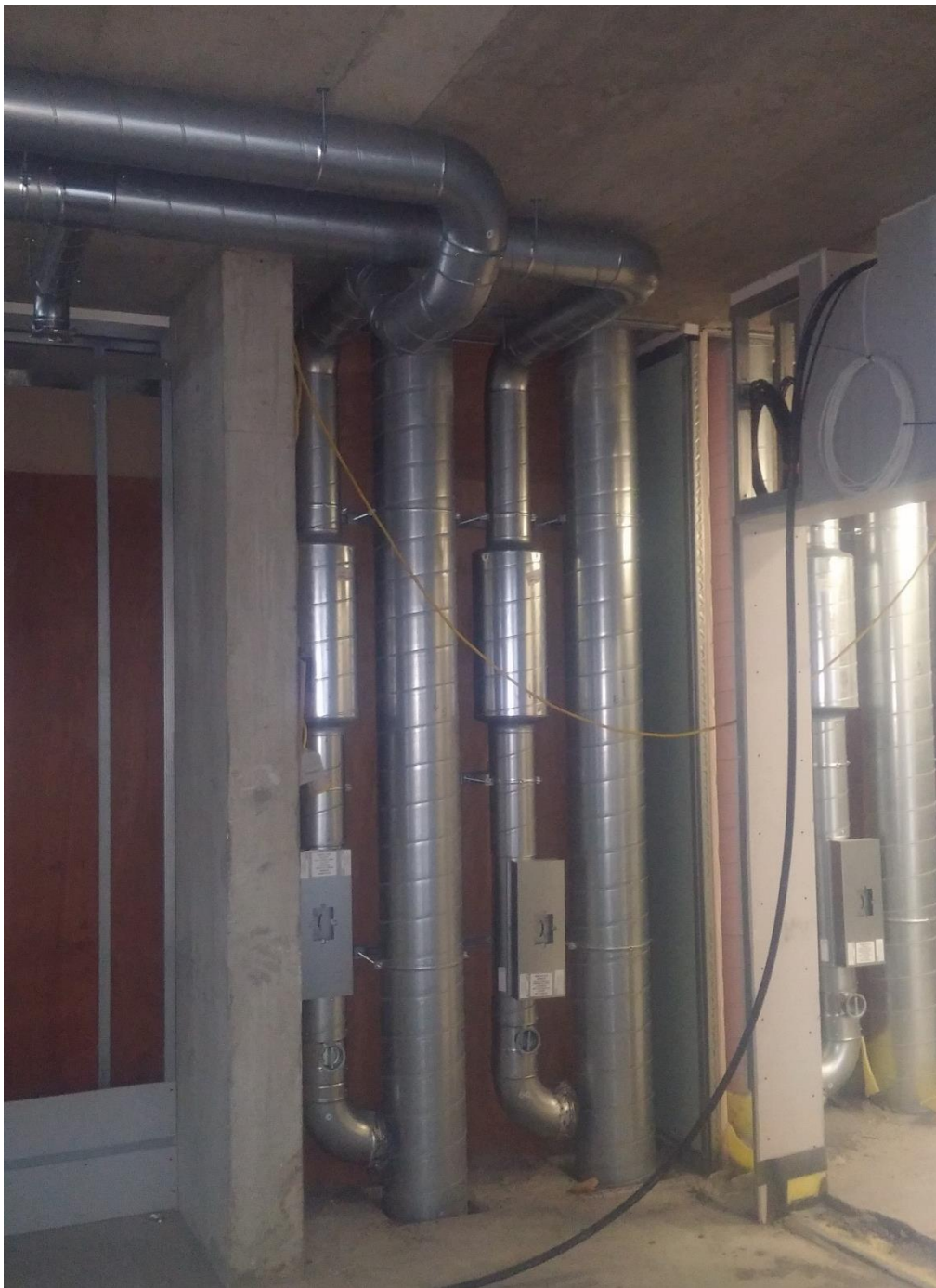
Ventilation riser, branch to apartment and damper arrangement.
