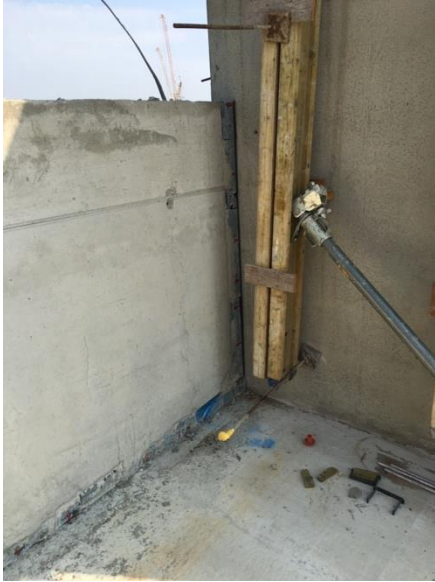
Image showing Halfen Thermal Breaks at parapet and adjoining junctions
