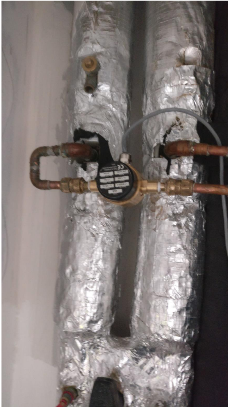
Remote differential pressure sensor for close control of variable speed LTHW pumping.
