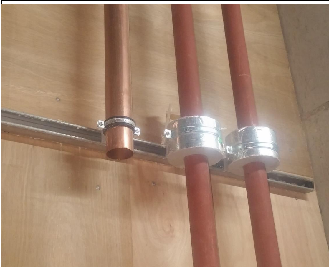
Thermally isolated pipe supports, during installation.
