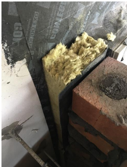
Image showing window closer installed
