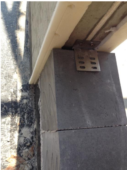
Inner leaf of AAC lightweight blockwork
