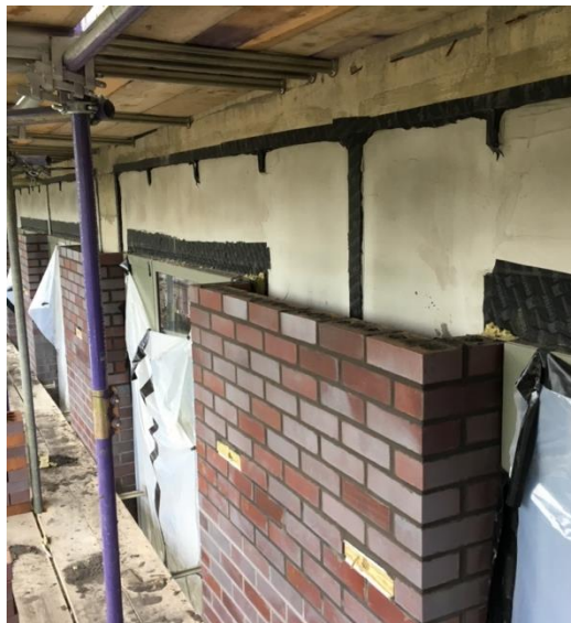
Image showing window closer installed
