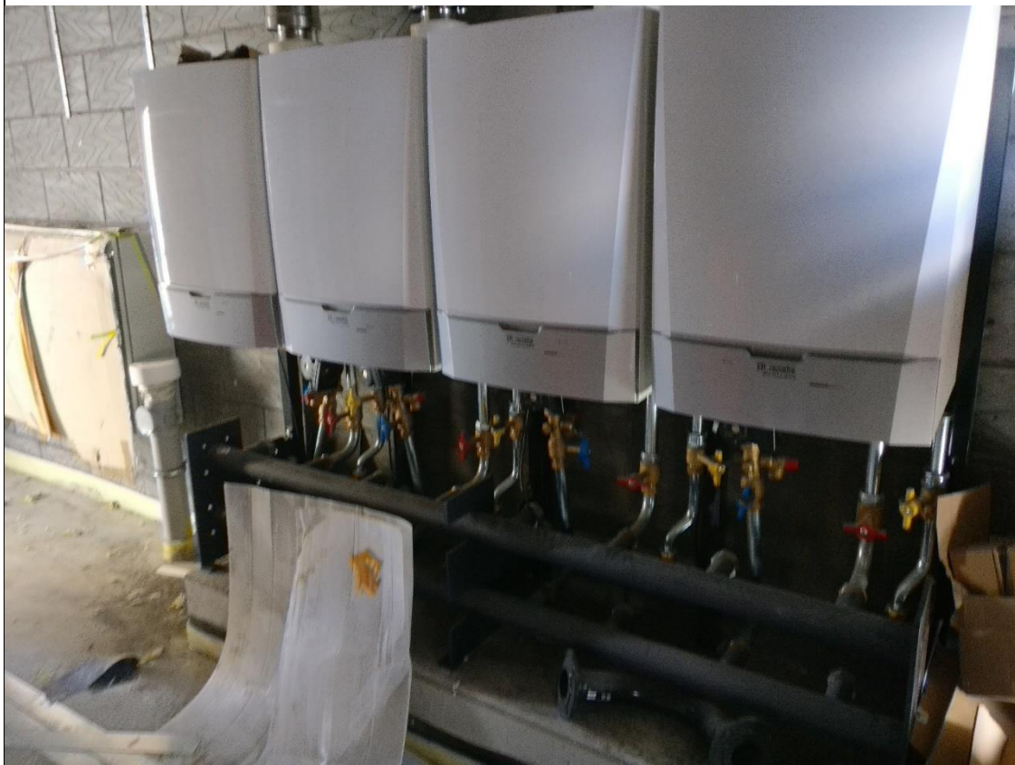
Thermally isolated pipe supports, during installation.
