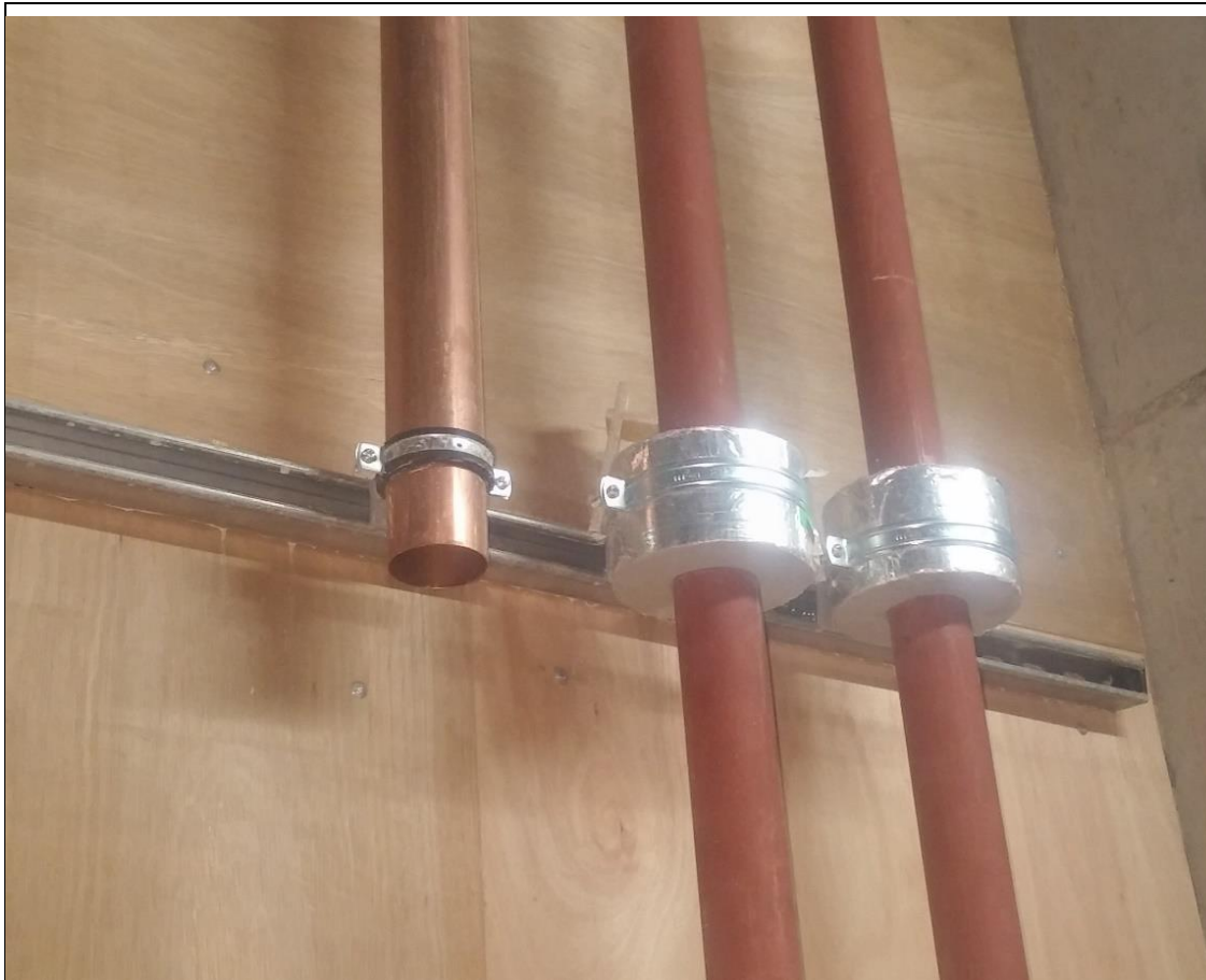
Thermally isolated pipe supports, during installation.
