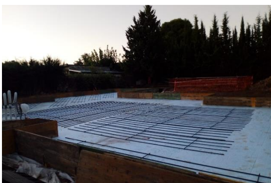
Basement floor insulation (Source: Metro7)
