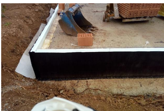
Ground wall insulation (Source: Metro7)
