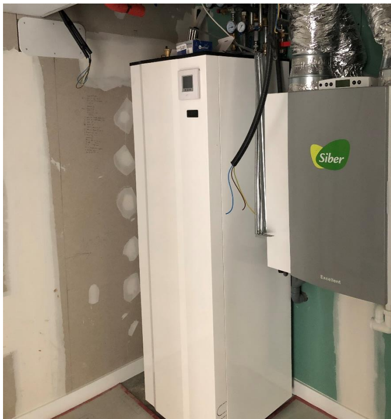
Water-to-Water Heat Pump in service room (Source: Metro7)
