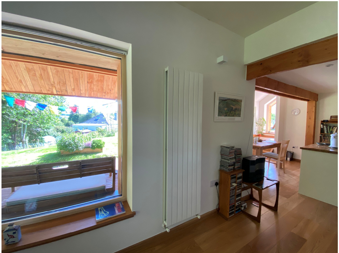
Radiator in living space – which provide heat from the thermal store when the wood burner is not being used.
