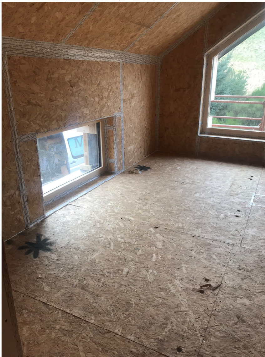
Taping to junctions of OSB and windows at first floor
