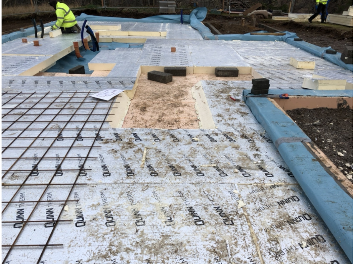
Under-slab insulation during construction.
