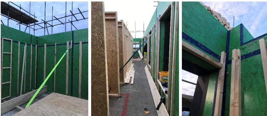
External walls built off-site and craned into place. There is full fill blown cellulose insulation between studs, and airtight board on the inside and a vent board on the outside.
