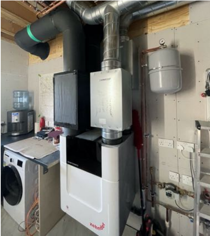
7.2.4 Ventilation unit in utility room
