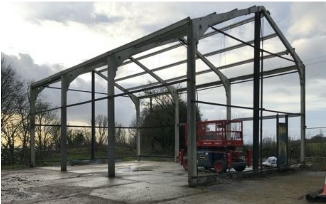
View of the concrete portals: once the cladding was removed the purlins were removed allowing the new timber frame to be inserted around the portals.
