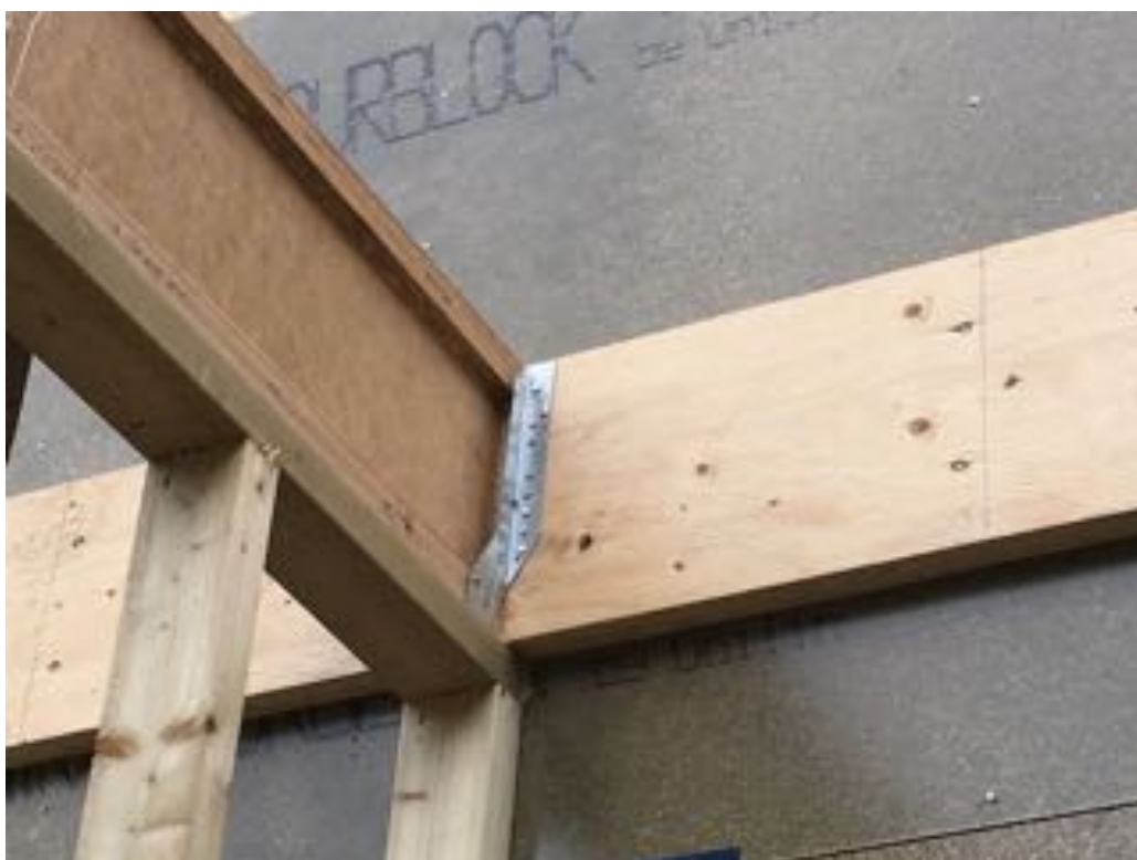
6.2 Internal image of 'rim board' to which first floor joists are hung.
