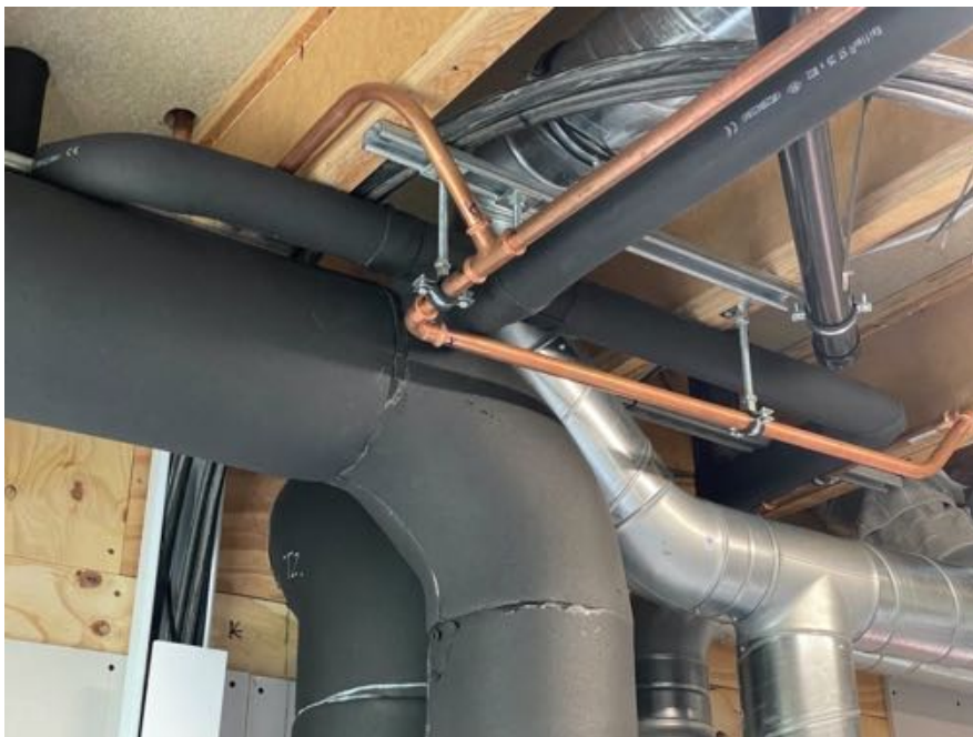
7.2.5 Insulated ductwork to exterior. Galvanised steel ductwork secured with rubber mounted brackets.
