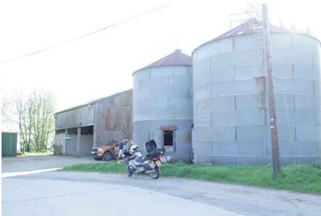
View from the north east of the original barn: the barn is clad with asbestos cement sheet and consists of 3 bays.
