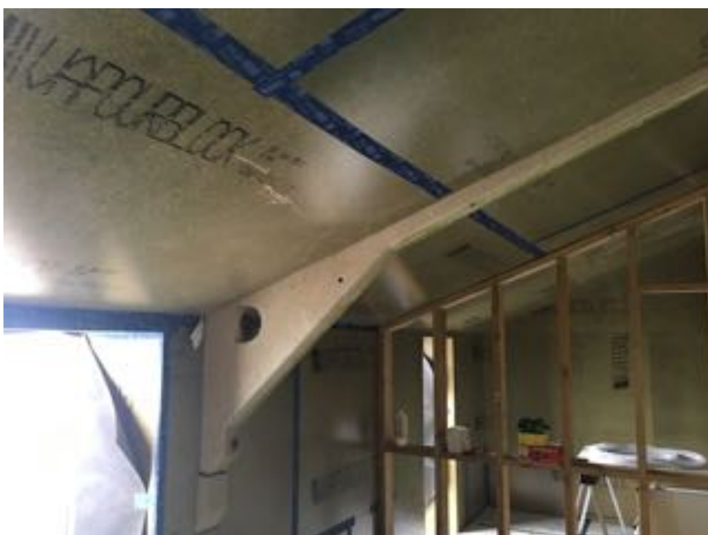
6.3 Internal image of airtight board to underside of roof with taped joints.
