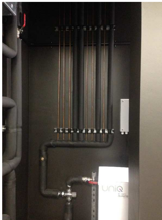
Sun amp phase change heat store and efficient small bore hot water distribution.
