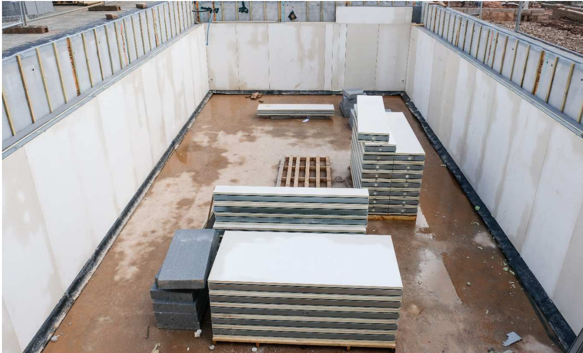
SIPS panels on walls of basement.
