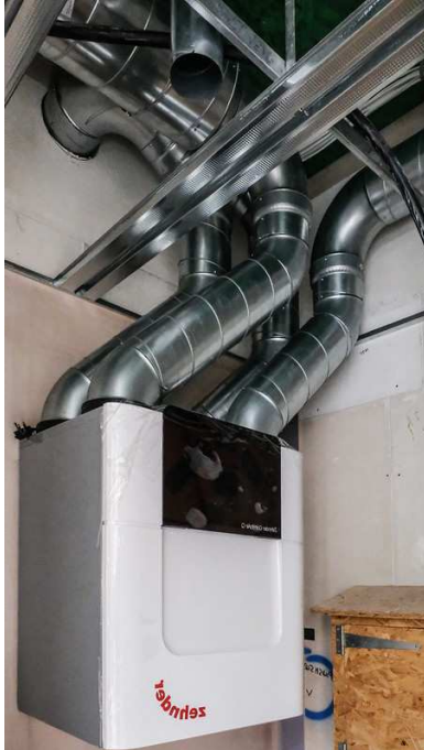
Zehnder ComfoAir Q450 installed prior to duct insulation being installed on intake/exhaust ductwork.
