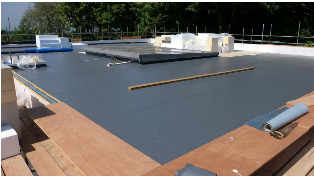
Vapour barrier on top of plywood deck
