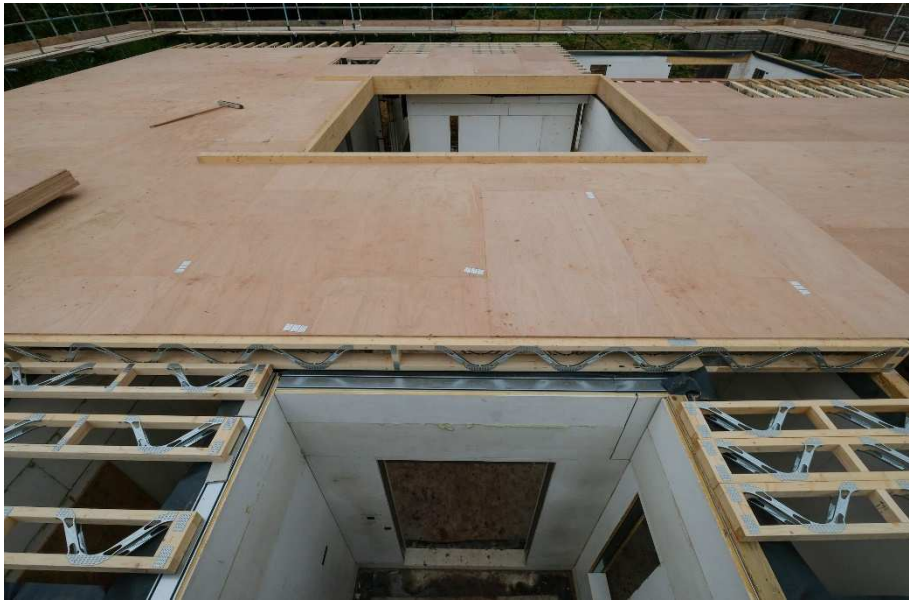
Roof plywood deck below insulation
