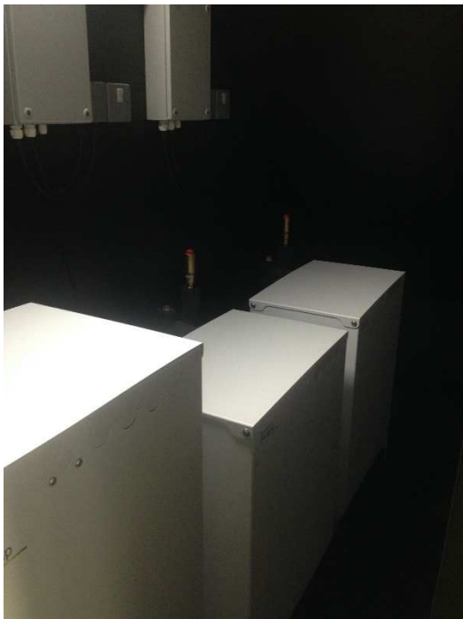
Sun amp phase change heat store and efficient small bore hot water distribution.
