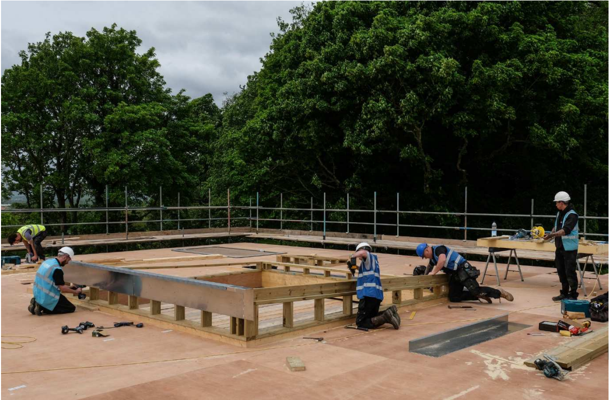
Large rooflight framing
