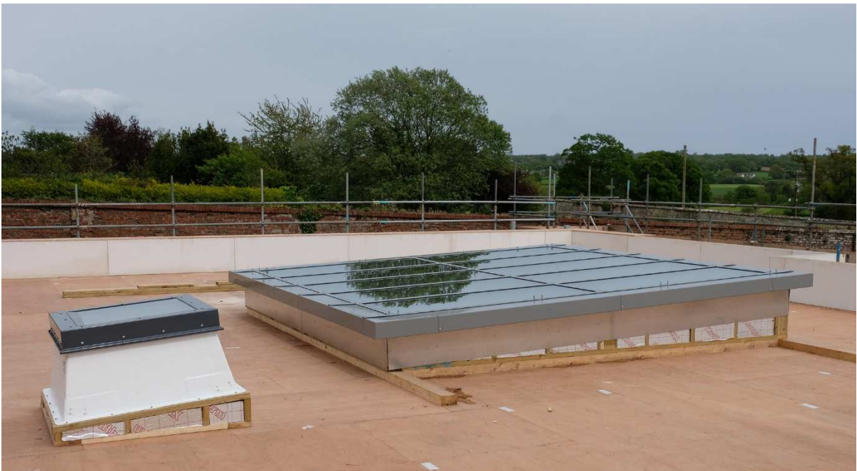
Roof light installation prior to insulation being added.
