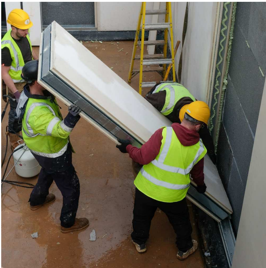
Basement walls, SIPS panel and insulation installation.
