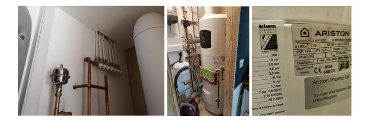
Heat supply is via an Ariston Nuos Plus Air Source Heat Pump with integral hot water cylinder (2001). This is mainly used for domestic hot water but also serves two towel radiators located in the bathrooms (one on each floor). The heat pump is located internally within the plant room, adjacent to an external wall for air intake via direct ducting.
