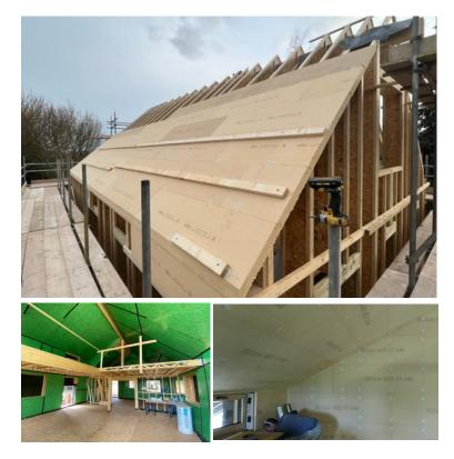
Both the wall and the roof are constructed from 300mm deep timber I-joists filled with Warmcel insulation (blown cellulose) with 80mm wood fibre insulation (Steico Special Dry) and timber cladding on battens applied externally. Internally, 12mm Pro-Passive OSB, with 40mm wood fibre (Steico Internal) with clay plaster. This enables a thermal bridge free junction at the eaves and verge.
