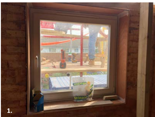
Photographs of window installation 1. Plywood box 2. Initial plaster base coat 3. Airtightness membrane and tape
