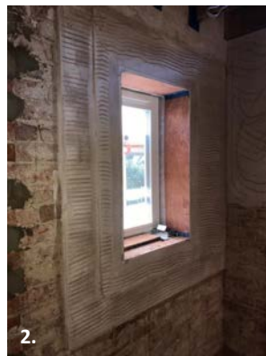
Photographs of window installation 1. Plywood box 2. Initial plaster base coat 3. Airtightness membrane and tape
