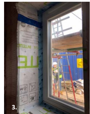
Photographs of window installation 1. Plywood box 2. Initial plaster base coat 3. Airtightness membrane and tape
