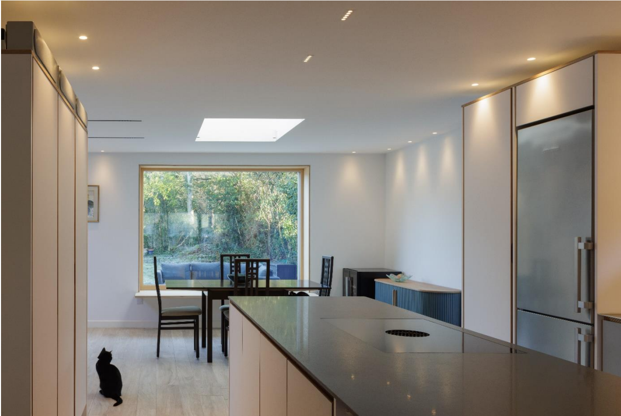
Interior view from the kitchen towards the dining area with the rooflights above to allow incoming air for the stack ventilation strategy
