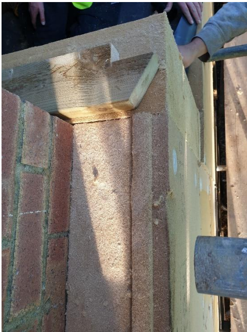
W-01 EWI Retrofit Wall and New Curtain Wall Junction
