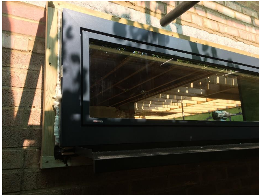
Window installed in existing brickwork wall
