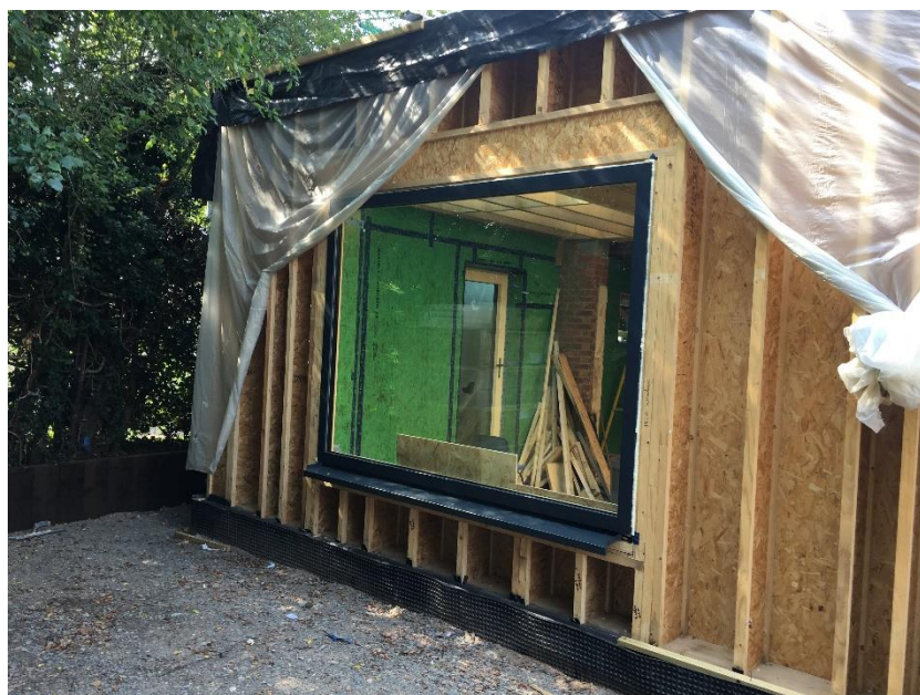
Window installed in rear extension timber frame
