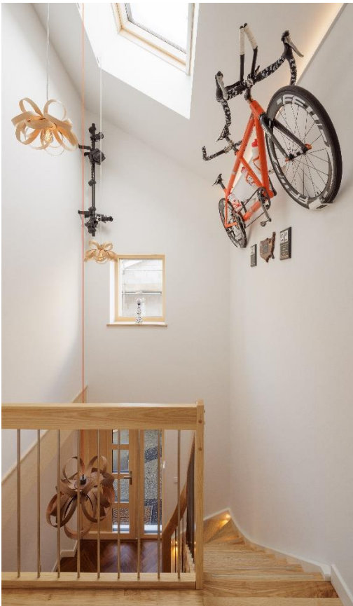
Interior view of vaulted stairwell with rooflight at the top to increase natural light in the centre of the property and allow the hot air to purge out of the building within the stack ventilation strategy
