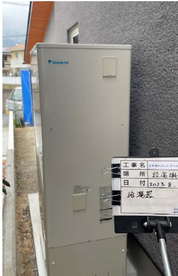
Hot water is provided by a heat pump hot water system and a 370 liter hot water storage tank. One room air conditioner is installed on the second floor for cooling and one room air conditioner on the first floor for heating.
