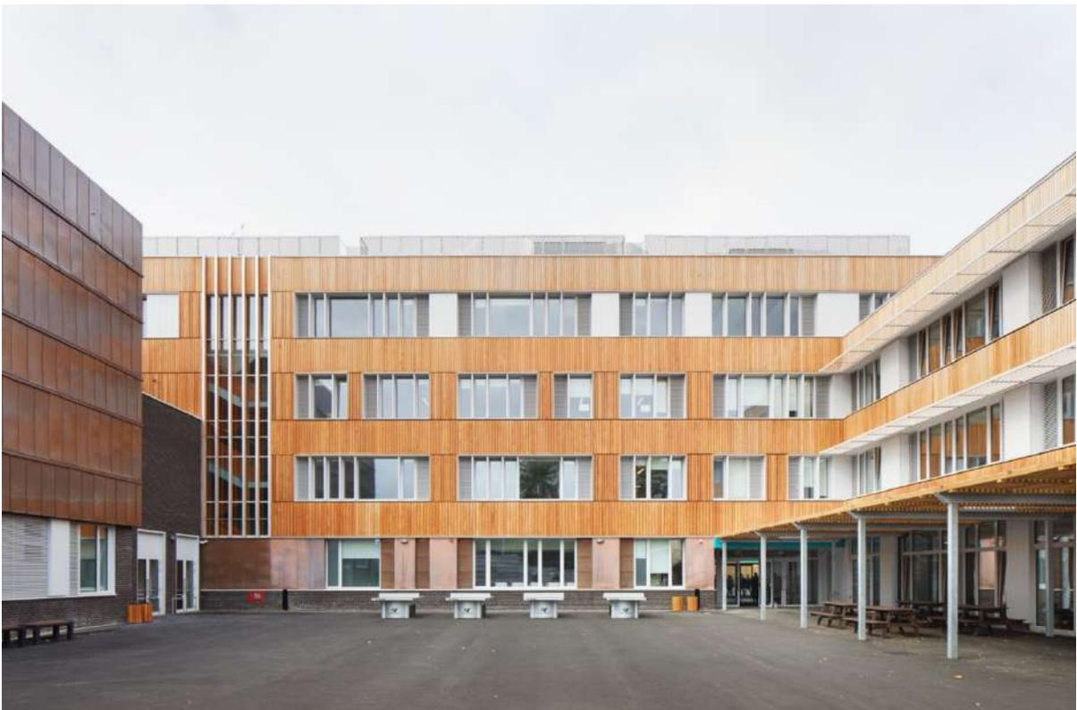
East elevation showing vertical shading on east façade, horizontal brise-soleil on south façades.
