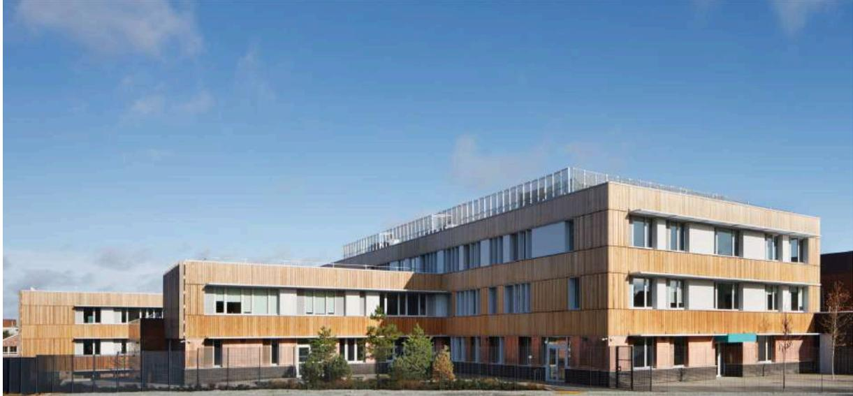
South elevations – teaching wings (left) span from central wing (right). MVHR units are located externally on the roof and are concealed behind metal mesh screening. The green canopy on south façade identifies the secondary rear entrance door from central spine. © Jack Hobhouse / Architype
