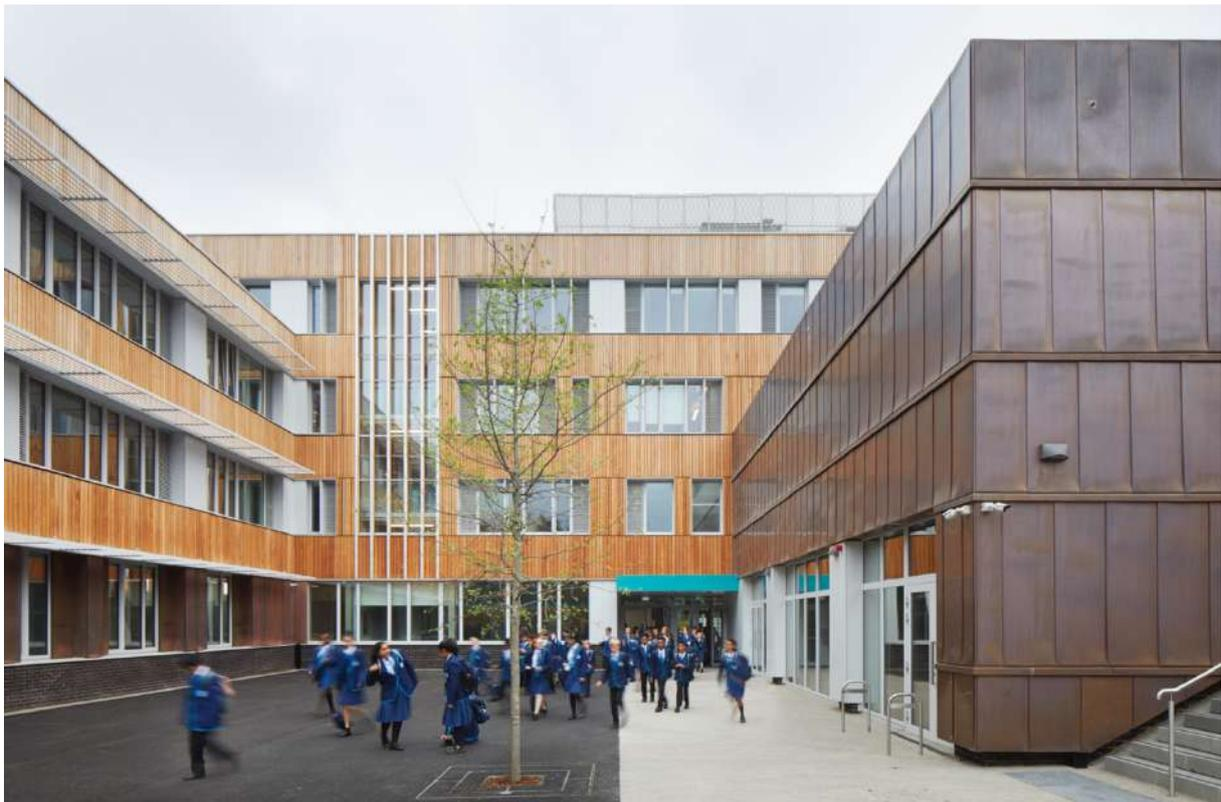
West elevation of central spine with vertical shading. Assembly Hall (with copper cladding) & front teaching wing (with brise-soleil) span from the central spine. | © Jack Hobhouse / Architype
