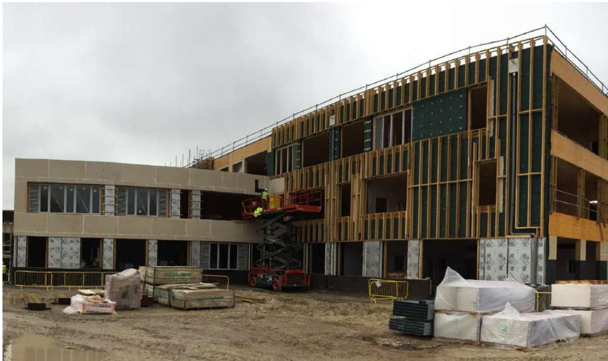
Photo showing framed JJI-joint structure (195 mm) fixed to glulam / timber frame infill. Zone was boarded (visible on left wing) before being fully-filled with blown insulation.
