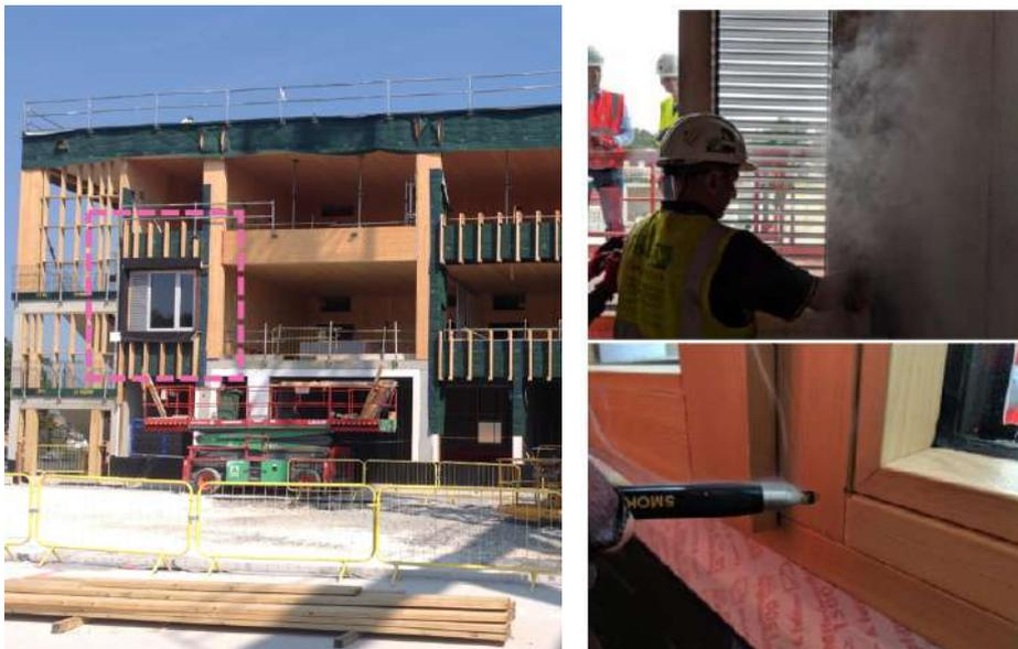
**Early-stage air tests** (above): An initial air test was carried out following installation of the first window (highlighted in pink) to check for problematic areas and confirm the installation quality was adequate. Further sectional air tests were undertaken before the final blow door test.
