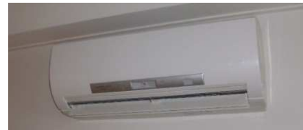
Figure 23 Heat pump indoor unit
