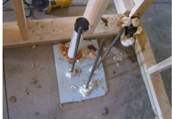
Figure 17 Spray foam at plumbing penetrations
