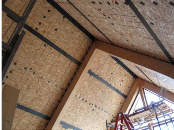
Figure 16 SIP flashing tape
