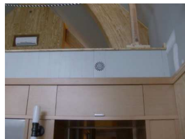
Figure 21 Supply air point in main room
