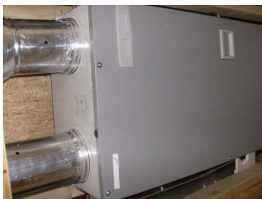
Figure 20 HRV in second floor cavity
