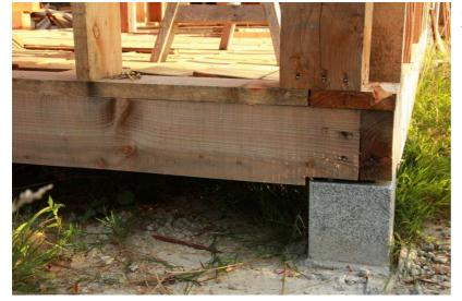
In the research of Japanese architecture, choose for L foundations some stones piles, the wood joist are fixed on it. It is also more easy to use natural insulation, between the joist with cellulose wadding of 160 mm. To complete insulation, I used VIP (vaccum insulation Pannel) because the ceiling height was already low. Those panels are really high insulation, with a lambda of 0.0077 W/m.K.
