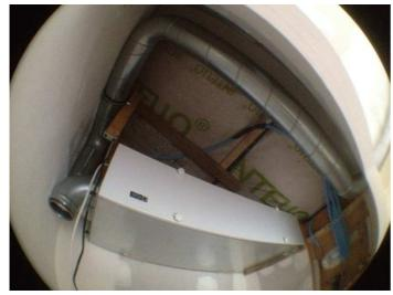
The ventilation hidden in a small technical ceiling : HELIOS KWL EC 220 PRO Phi certified : 88% 0.4 Wh/m3
