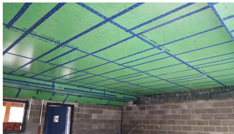
Figure 9 Air tight OSB Board in top floor ceiling taped with proprietary air tightness tape at junctions
