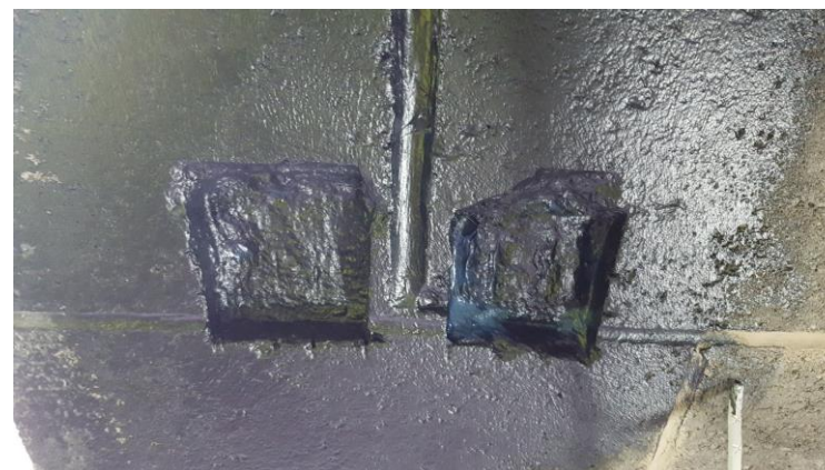
Figure 10 Blowerproof paint applied to socket/wiring cutouts in blockwork. Paint is blue when applied and black when dried and air tight.
