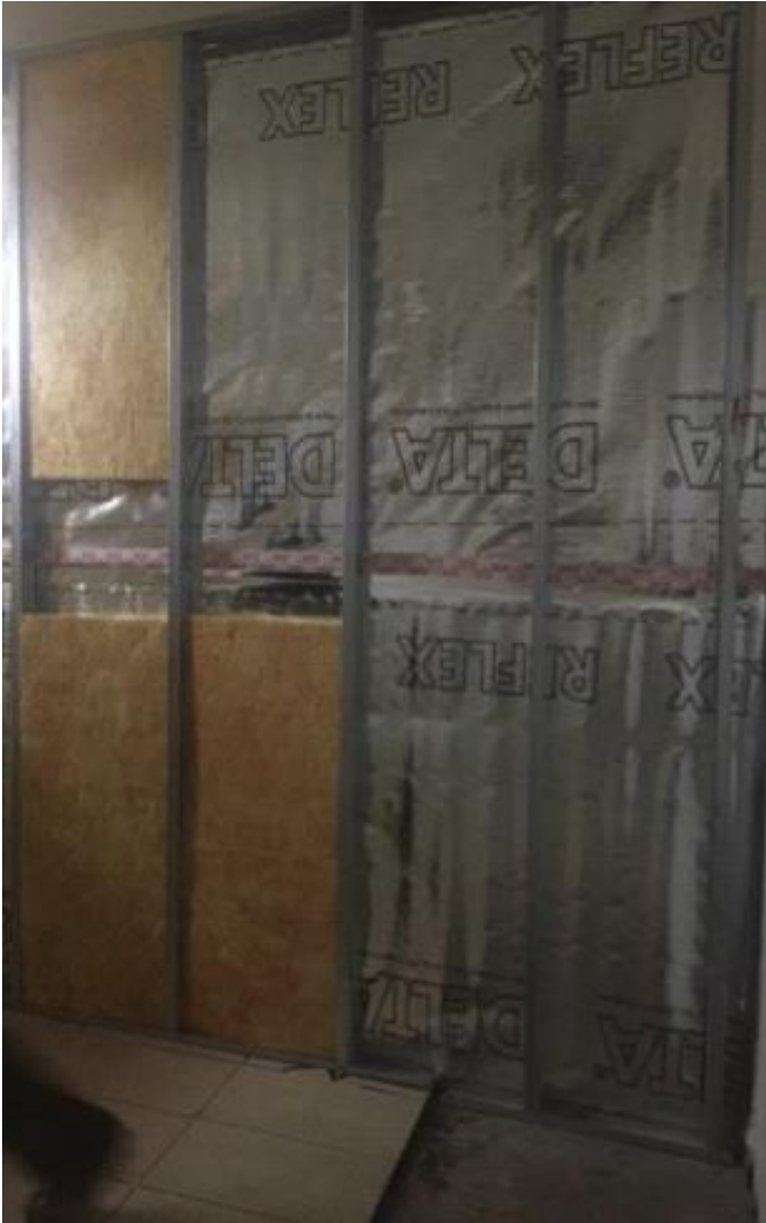
Thermal Envelope – Wall's inside view with insulation and airtightness membrane
