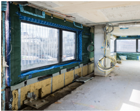
Before Panel Supports Sealed
