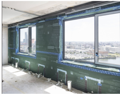
After Panel Supports Sealed
