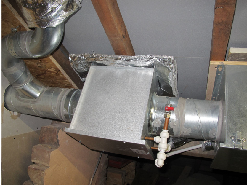
Duct heater fed from Condensing Combi Boiler
