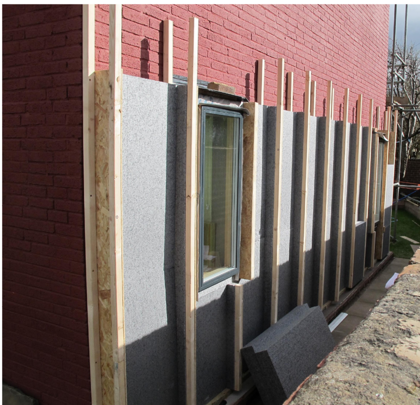
External insulation being installed
