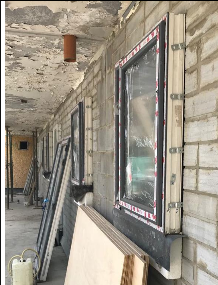
External window fitted with insulated EPS support bolted to walls.
