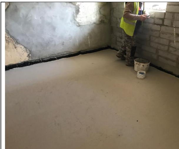
Floor wall seal with airtightness liquid applied membrane
