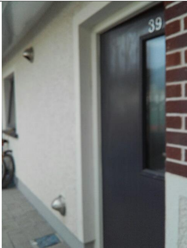
Supply and extract air ducting outlets on outside wall
