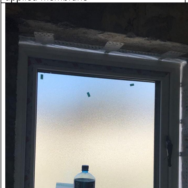
Airtightness taping around windows. Note fixings are taped.
