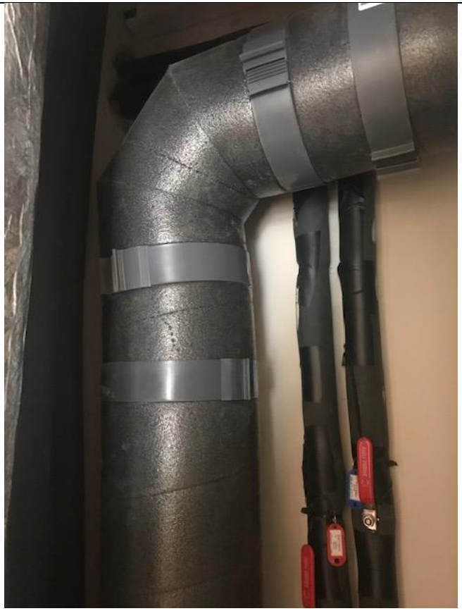
Insulated ducting with supports
