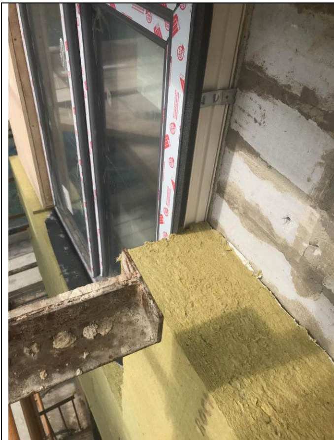
Junction showing the External insulation abutting the External Window jamb
