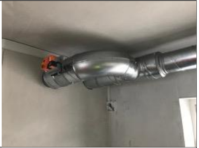
Extract ducting to kitchen area
