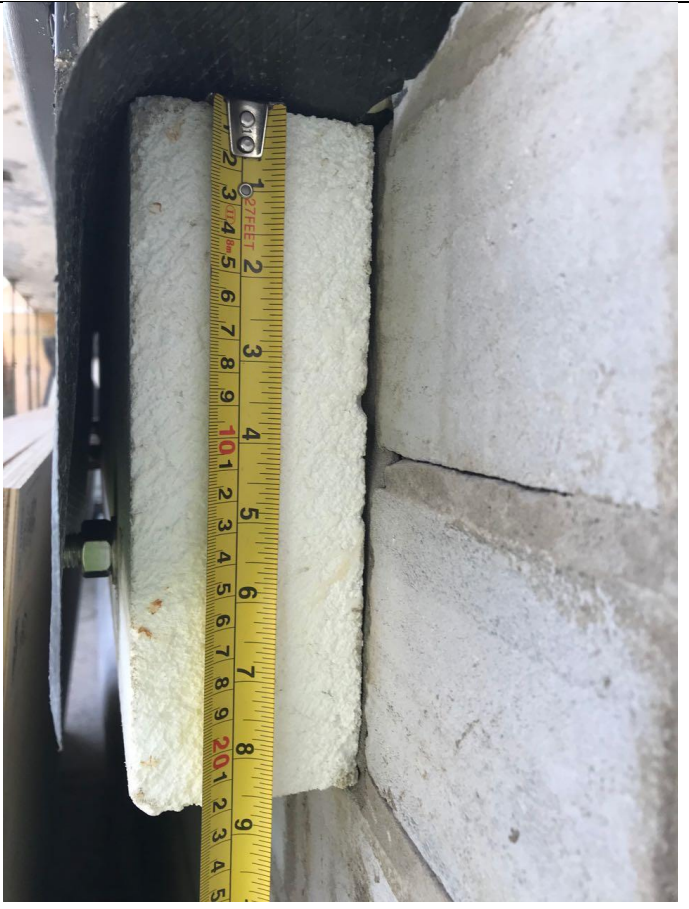
CompacFoam EPS external window support.
