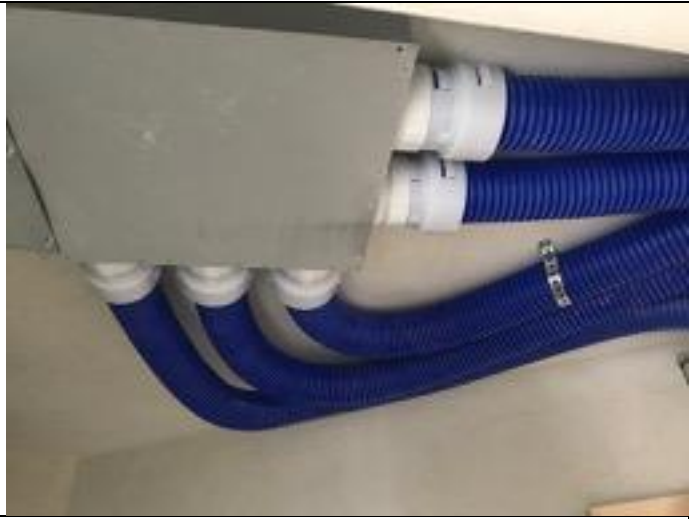
Supply air ducting with manifold
