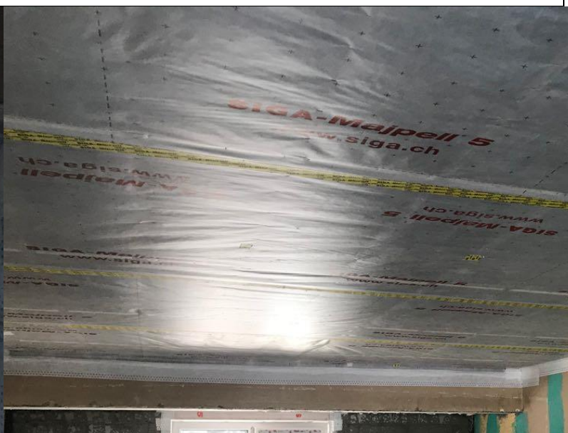
Example of Ceiling membrane taped
