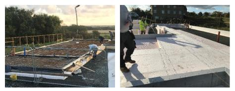
Insulation below the slab reduces thermal bridges the connection around between the timber frame and the foundations. "Floating Floor" insulation the slab further over reduced any losses through the sole plate.
