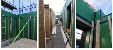
External walls built off-site and craned into place. There is full fill bllown cellulose insulation between studs, and airtight board on the inside and a vent board on the outside.
